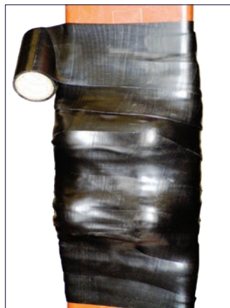
Figure 20: Insulation with half-lapped tape
