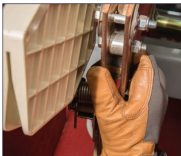
Figure 42: Disengage switch blades
