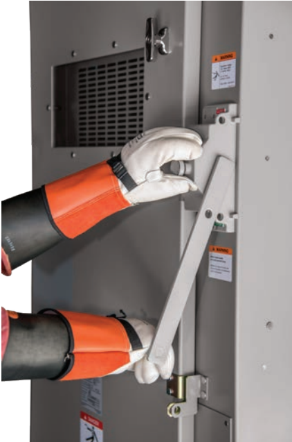
Figure 29: Operation of the load-interrupter switch
