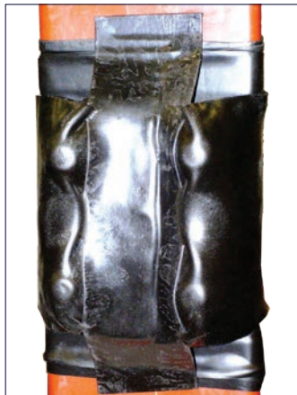
Figure 19: Installation of mastic pads
