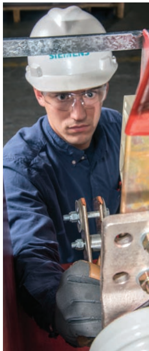
Figure 44: Reconnect pushrods
