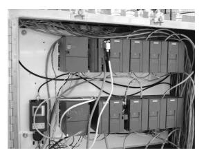
As it turns out, the visual inspection provided the most significant information for the two PROFIBUS DP networks. At installation, several PROFIBUS DP wiring guidelines had been contravened: cable types were mixed and powered terminators were not used. However, since the network was running at 9600 baud and the copper wires were going less than 100 meters, these violations had little or no impact on the error rate.<sup>5</sup>
