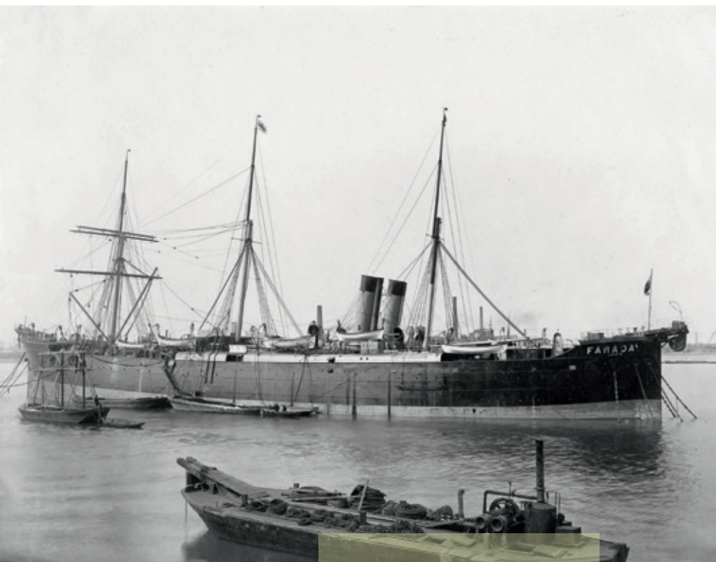
Setting the standard for laying submarine cables – the cable steamer Faraday , 1874
