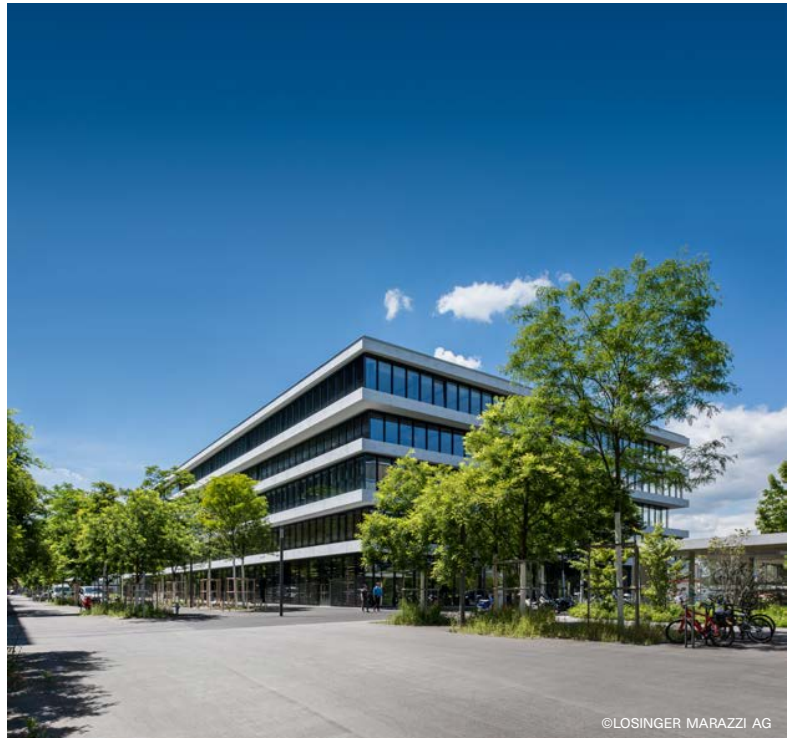
Twist Again in WankdorfCity, Bern, is the first SNBS 2.0 certified building in Switzerland
