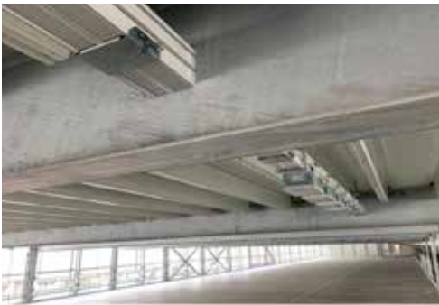
Abb. 7/4: Cutouts in the steel structure of a parking level for a busbar trunking system
