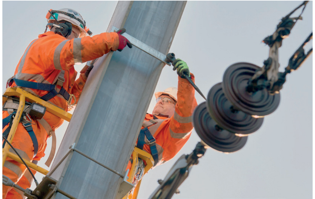
East Coast Power Supply Upgrade: Siemens Mobility is part of the alliance responsible for upgrading equipment on this key artery. Courtesy Network Rail
