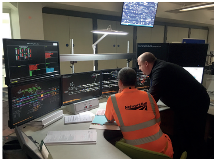
New workstation at Manchester Rail Operating Centre: Siemens Rail Automation's Dynamic Route Setting product has been installed here. Courtesy Network Rail
