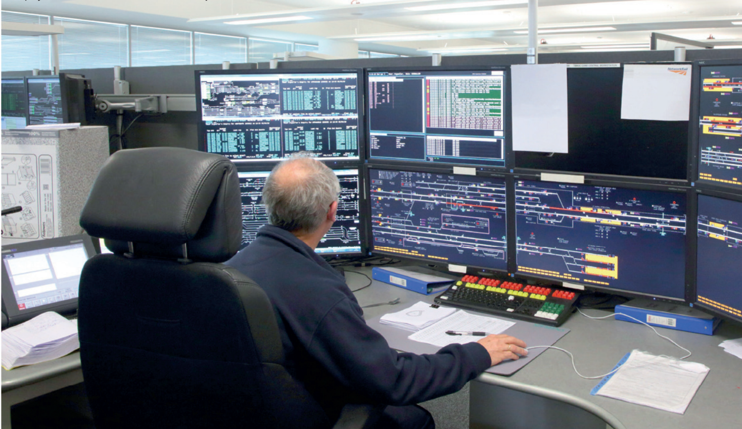
Central core: this is the workstation at Three Bridges for the Thameslink line through Blackfriars. ATO information is displayed on one of the side screens. Jamie Squibbs
