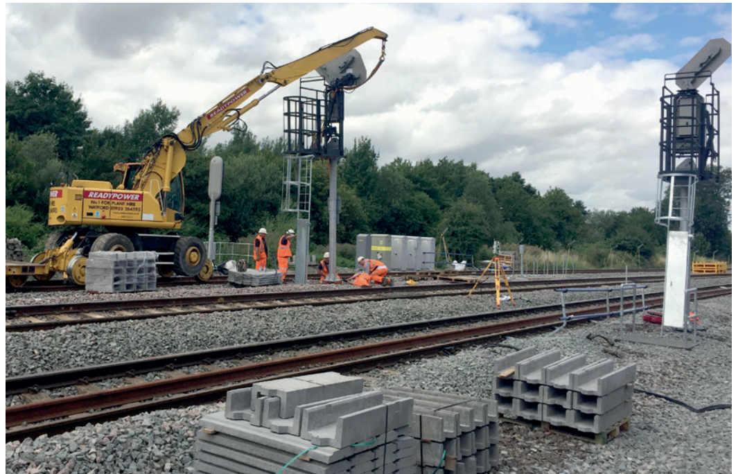
New equipment: a roadrunner assists a team installing a new signal post at Banbury in 2016.
