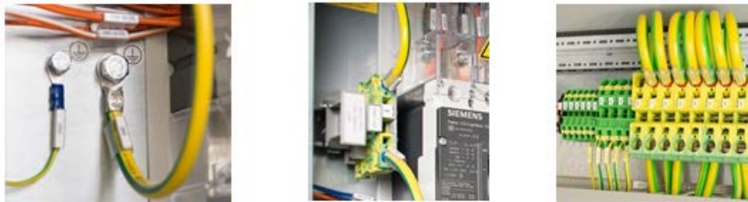
Figure 6-45 Examples: Components of the protective bonding circuit
