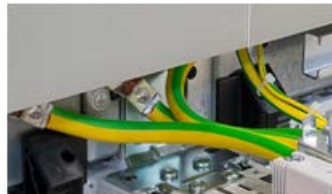
Figure 6-48 Example: Protective conductor with GREEN-AND-YELLOW insulation
