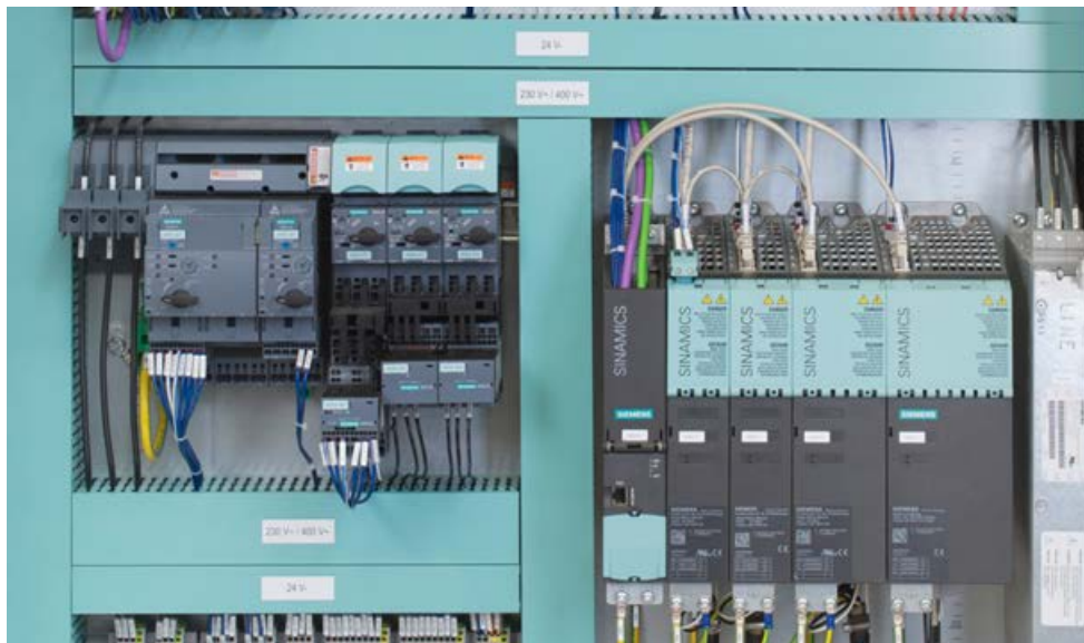
Figure 6-65 Example: Separate routing of 24 V and 230 V/400 V circuits
