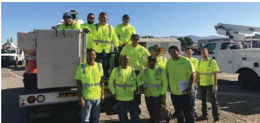
Teams of Siemens Mobility electricians installed 40,952 LED streetlights for the 11 participating jurisdictions involved in the Western Riverside Council of Governments' retrofit program. At the height of the activity, Siemens Mobility installed almost 6,000 lights in one month.
