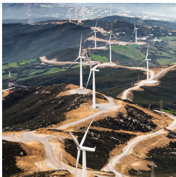
Wind power plant
