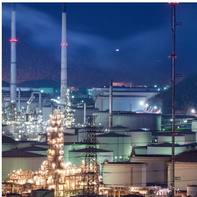
Industrial application: Refinery
