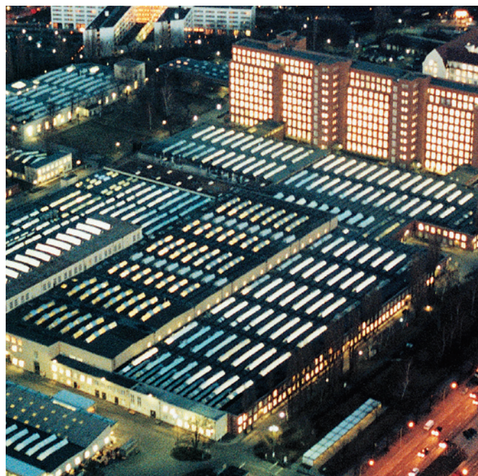
Switchgear Factory, Berlin
