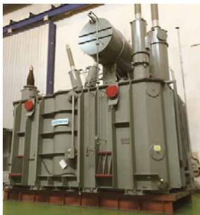
500-kV single-phase autotransformer in the test bay
