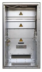
Fig. 200: Switching-device compartment without ventilation duct
