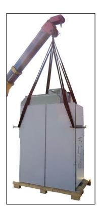
✓ The panel is prepared for craning with crane rods.
