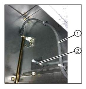
Fig. 163: Optical sensor (2) and connecting cable (1), for example, in the switching-device compartment
