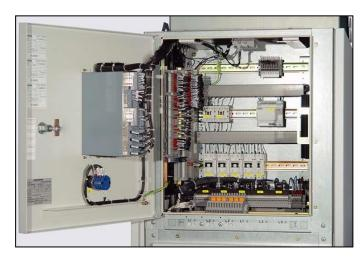
Fig. 230: Inside view of the low-voltage compartment as an example
