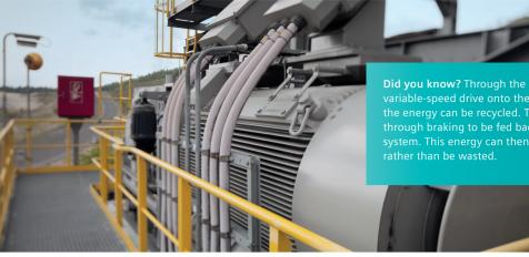
**Did you know?** Through the installation of a regenerative variable-speed drive onto the hoist system or a downhill conveyor, the energy can be recycled. The drive allows the energy created through braking to be fed back into the main energy supply system. This energy can then be used again to power the hoist, rather than be wasted.
