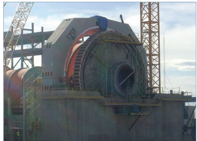
Figure 4 – 38 ft SAG mill with GMD in installation phase; rotor poles bolted onto the mill flange and stator shifted back to the maintenance/installation position
