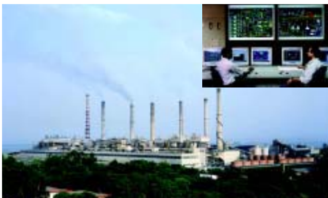
Hindalco Renusagar, trusted our Power Generation division for the revamp of their units 3 & 4.
