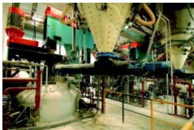
A&D successfully commissioned equipment for a large DCS system at Asian Paints' biggest water based paint plant in Tamil Nadu.
