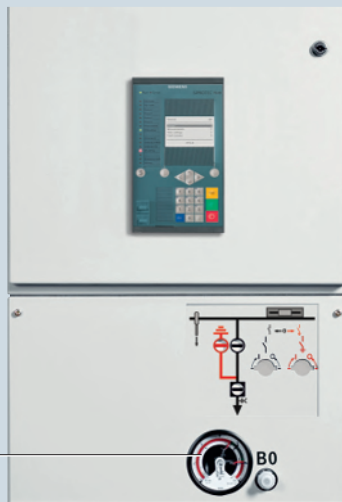
Gas pressure manometer (1) for circuit breaker housing (arranged at the panel front)
