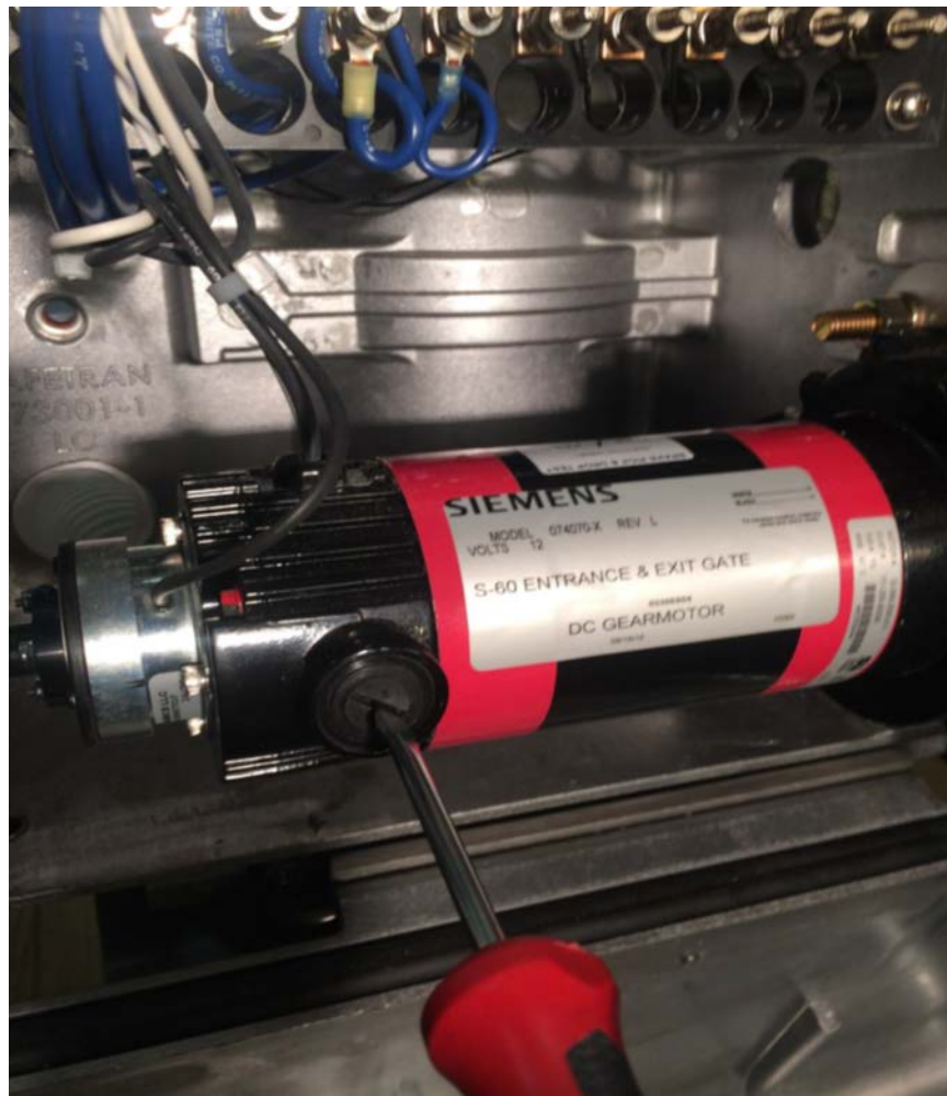
Figure 5-4 Removing Outside Brush from Motor
