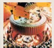
Siemens installs the first of 18 Itaipu generator rotors, with a power of 823.6 MVA.
