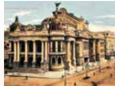
Siemens installs the first diesel-electric unit at the Municipal Theater of Rio de Janeiro.
