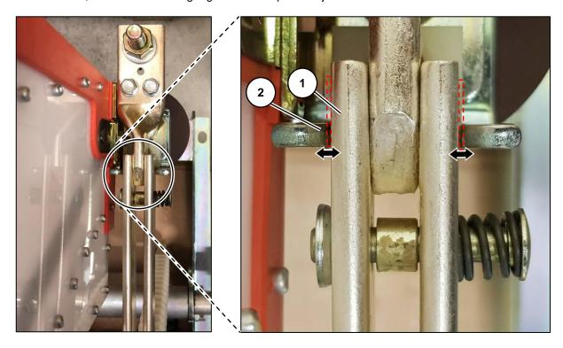
Fig. 80: Minimum distance between the main contact blade (closed position) and the edges of the notch
