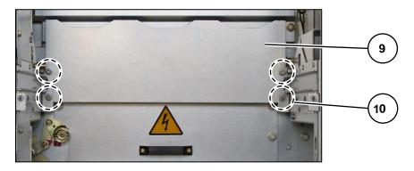
Fig. 231: 4 bolted joints on protection plate of switching-device compartment
