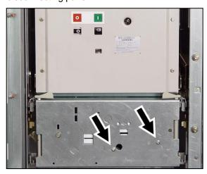
Fig. 276: Front view of withdrawable circuit-breaker
