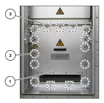
Fig. 233: 15 bolted joints on partition
