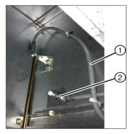
Fig. 127: Optical sensor (2) and connecting cable (1), for example in the switching-device compartment
