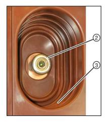
Fig. 272: Bushings in switching-device compartment
