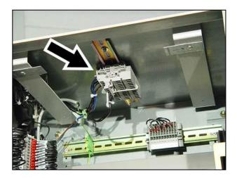
Fig. 222: Inside view of the low-voltage compartment with terminal block
