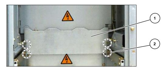
Fig. 163: 4 bolted joints on protection plate
