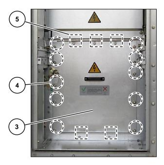
Fig. 137: All panel versions except for contactor panels with panel width 435 mm and switch-disconnector panel:15 bolted joints on partition
