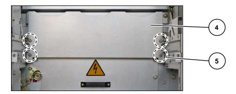
Fig. 234: 4 bolted joints on protection plate of switching-device compartment
