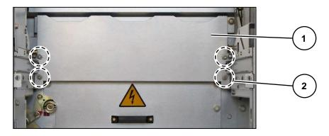
Fig. 136: 4 bolted joints on protection plate of switching-device compartment.
