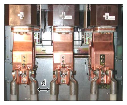
Fig. 206: Detail view: Minimum distance between cable lugs of adjacent phases
