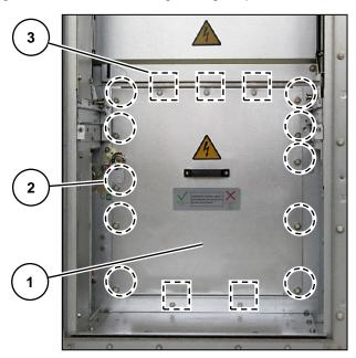
Fig. 224: All panel versions except for contactor panels with panel width 435 mm and switch-disconnector panel: 15 bolted joints on partition
