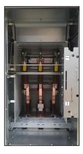
Fig. 135:Switch-disconnector panel only: Switching-device / connection compartment accessible
