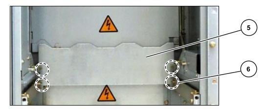
Fig. 247: 4 bolted joints of protection plate
