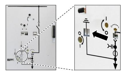
Fig. 193: Position indicator of feeder earthing switch on high-voltage door
