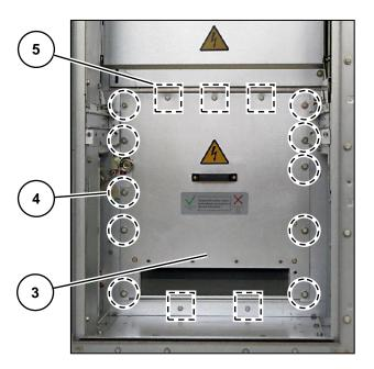
Fig. 159: 15 bolted joints on partition
