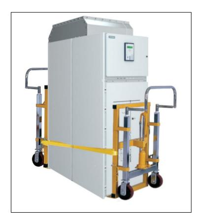
Fig. 42: The panel placed on hydraulic lifter
