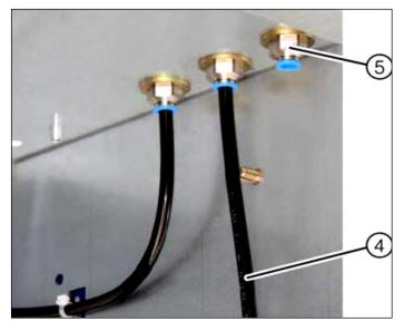
Fig. 129: Overpressure monitors (5) and tubes (4), for example in the switching-device compartment
