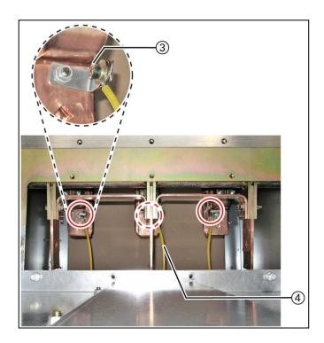
Fig. 251: 3 bolted joints at the cable connections (central joint covered)
