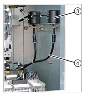
Fig. 128: Overpressure monitors (3) and tubes (4) in the low-voltage compartment
