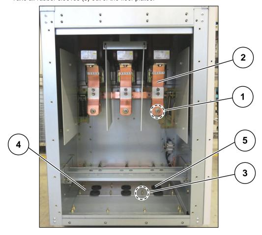
Fig. 195: Connection compartment, view from the rear side of the panel (installation of insulating plates only for  $U_r = 17.5 \text{ kV}$ )
