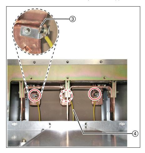
Fig. 181: Bolted joints at the cable connections (central joint covered)
