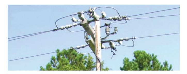
The Topper series of switches takes its name from the original Topper switch, a pole top-only design of unequalled compactness, ease of installation and unique synchronized operation. The same proven hot parts are used on all Topper styles. The Topper series is conservatively rated and has superior fault close, three-second, continuous and loadbreak ratings.
