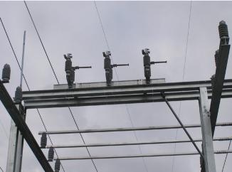
The Topper series switches can be customized to fit substation structures. The switches are designed to be installed in existing or new substations. The Topper is a fully factory adjusted, unitized switch which reduces installation time and costs.
