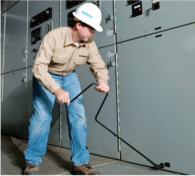
Before: Original hand crank racking, commonly used on GM switchgear, requires the operator to stand in front of the cubicle.
