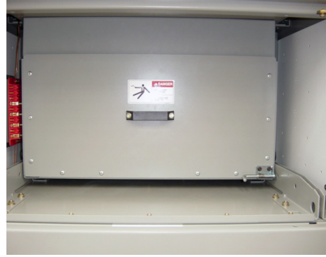
B. Handle/interlock bar retracted to allow rollout tray to be withdrawn.
