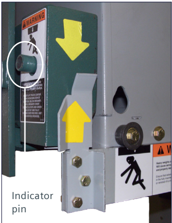
Figure 41: Lift truck engaged - note position of indicator pin
