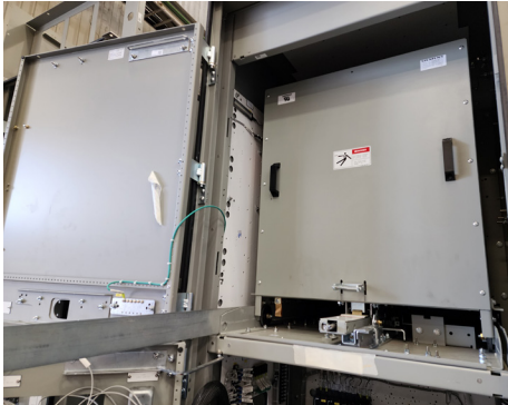
C. Extension rail being inserted.
