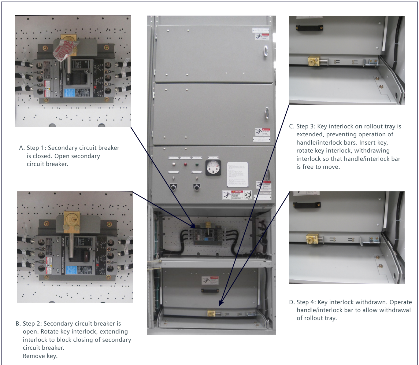
Figure 32: CPT fuse rollout tray with key interlocks
