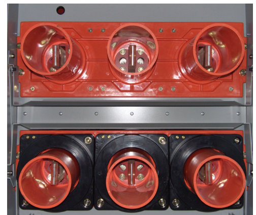
Figure 33: Type MD CTs installed on lower disconnect bushings (CT barrier removed for photo)
