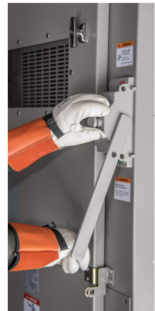
Figure 61: Operation of the load-interrupter switch
