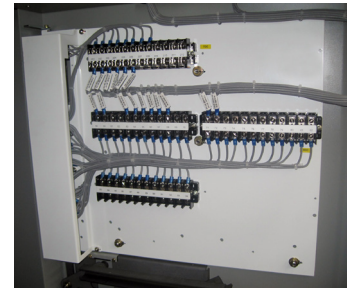
Figure 36: MOC and TOC switches
