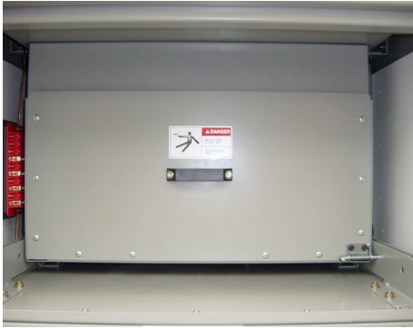
A. VT rollout tray in CONNECTED position. Handle/interlock bar fully extended to secure VT rollout tray in cell.
