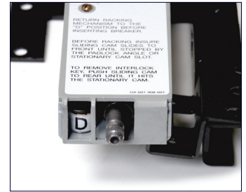
Figure 44: Racking mechanism shown in DISCONNECT position
