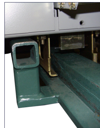
Figure 50: Alignment of lift truck with circuit breaker
