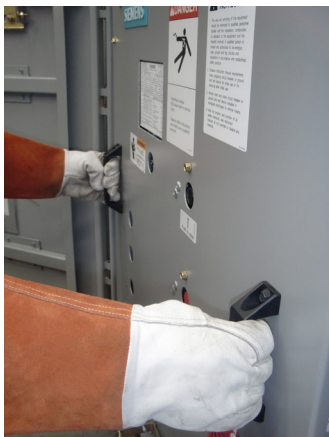
Figure 39: Removal of a circuit breaker
