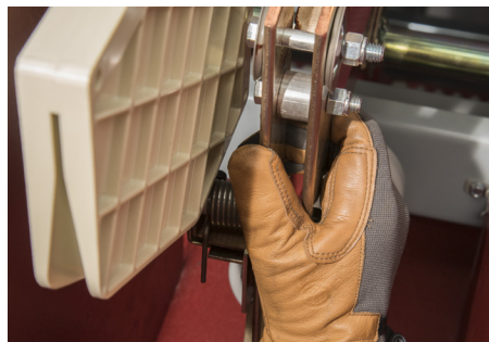
Figure 64: Disengage switch blades
