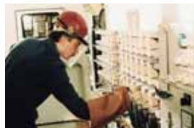
Fig. 3.2.4 – Actuating LV HRC fuse links under load
