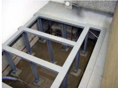
Fig. 38: Frame construction with longitudinal girders
