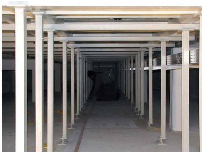
Fig. 39: Frame construction with longitudinal girders (cable basement)
