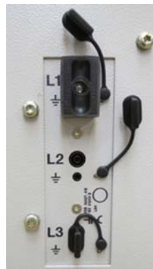
Fig. 17: Verification of safe isolation from supply (LRM system)
