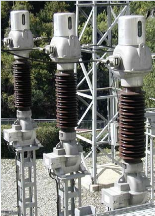
Fig. 50: 550 kV oil-immersed combined instrument transformers
