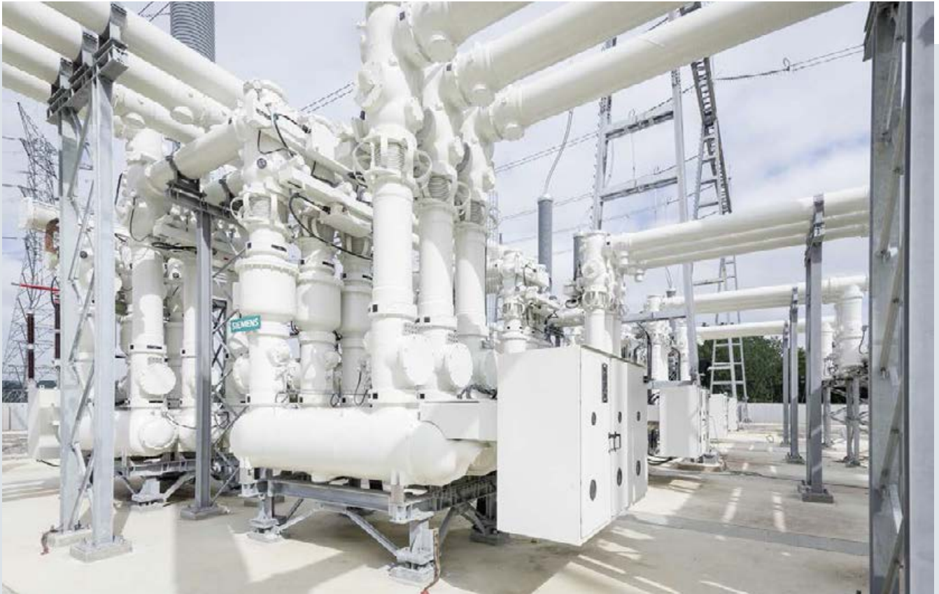
Fig. 92: 8DQ1 switchgear for a rated voltage of 420 kV
