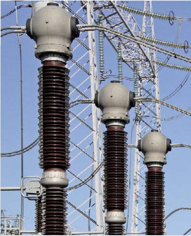
Fig. 44: 420 kV gas-insulated current transformers
