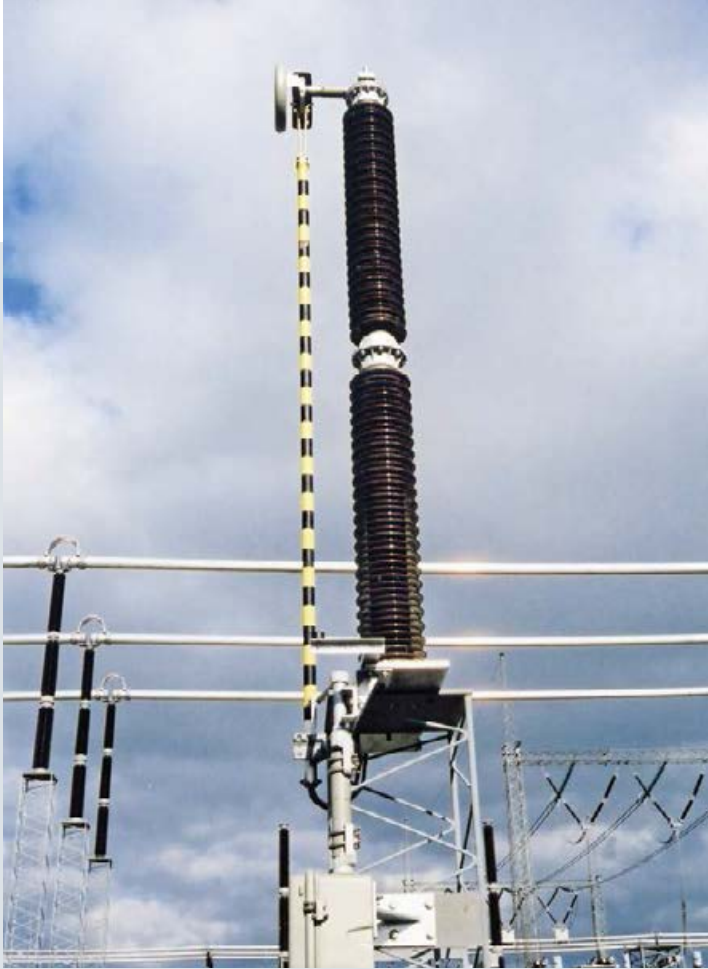
Fig. 30: Free-standing earthing switch
