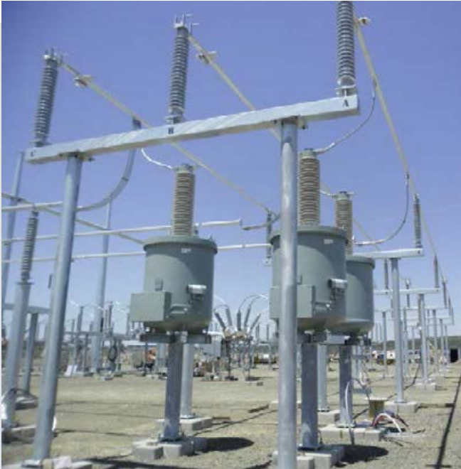
Fig. 61: 145 kV power VT for AIS
