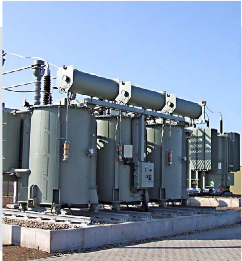
Fig. 70: Variable shunt reactor
