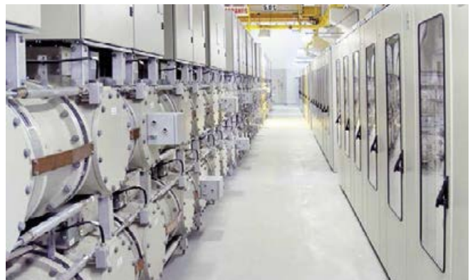
Fig. 87: 8DN8 GIS for a rated voltage of 145 kV
