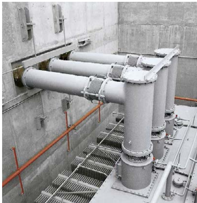
Fig. 98: Transformer termination
