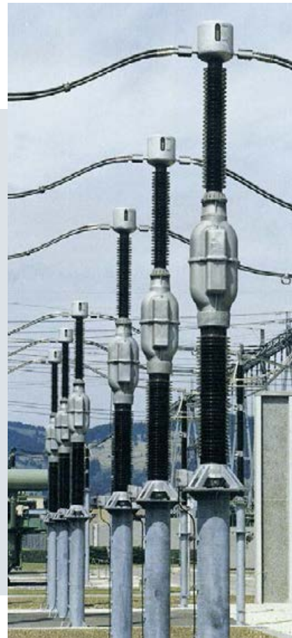
Fig. 49: 420 kV oil-paper-insulated inductive voltage transformers
