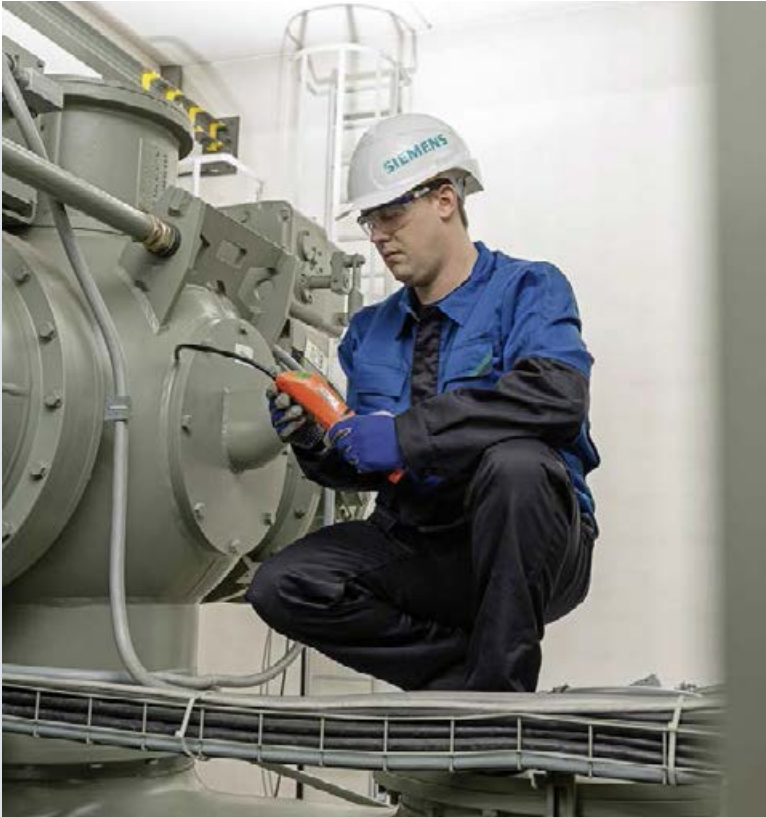
Fig. 105: SF 6 tightness test
