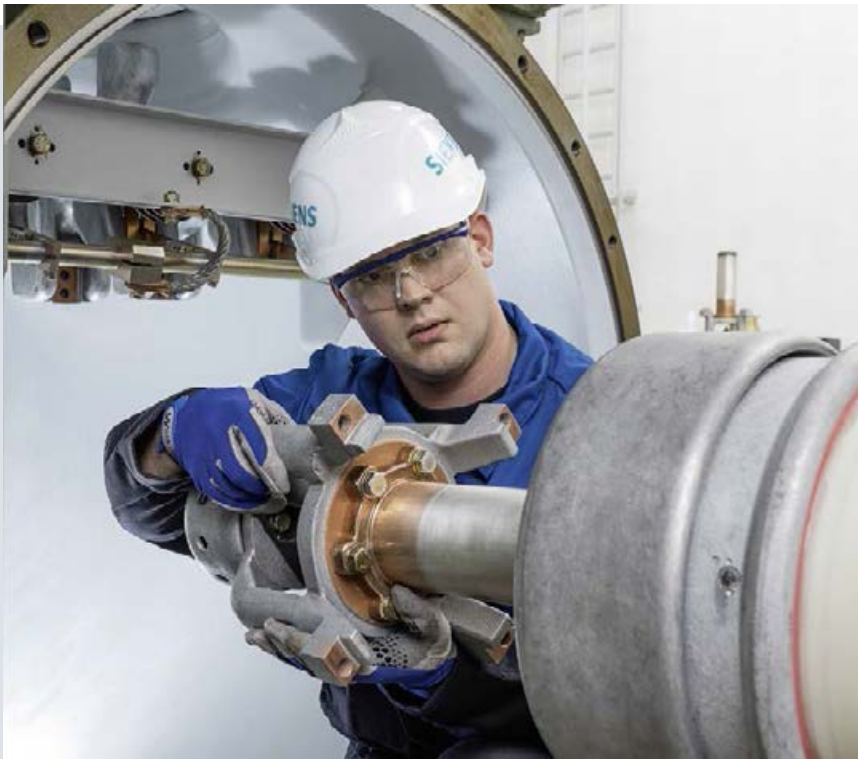
Fig. 106: Contact check of the interrupter unit
