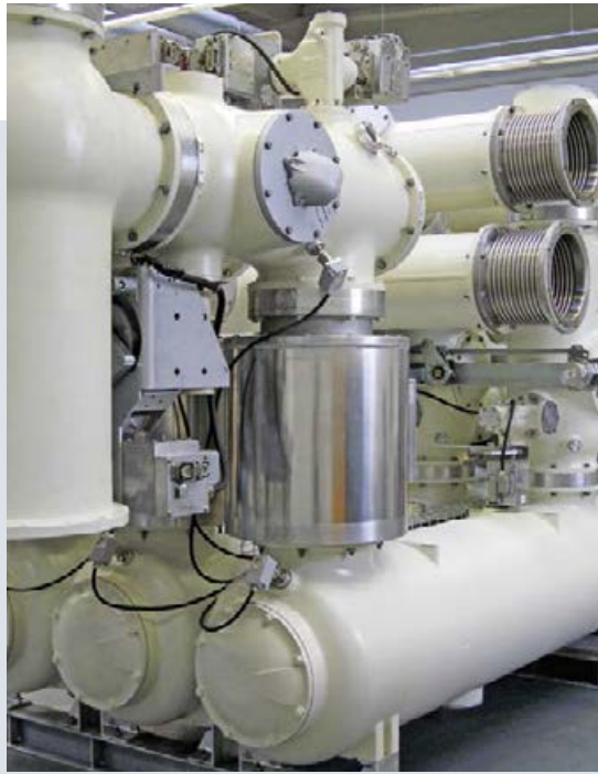
Fig. 58: 420 kV core-in-air current transformer for GIS
