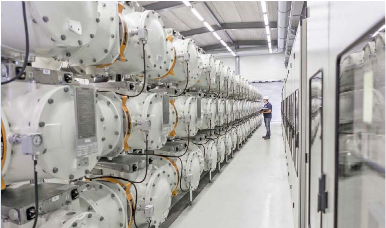
Fig. 83: 8DN8 GIS for a rated voltage of 110 kV
