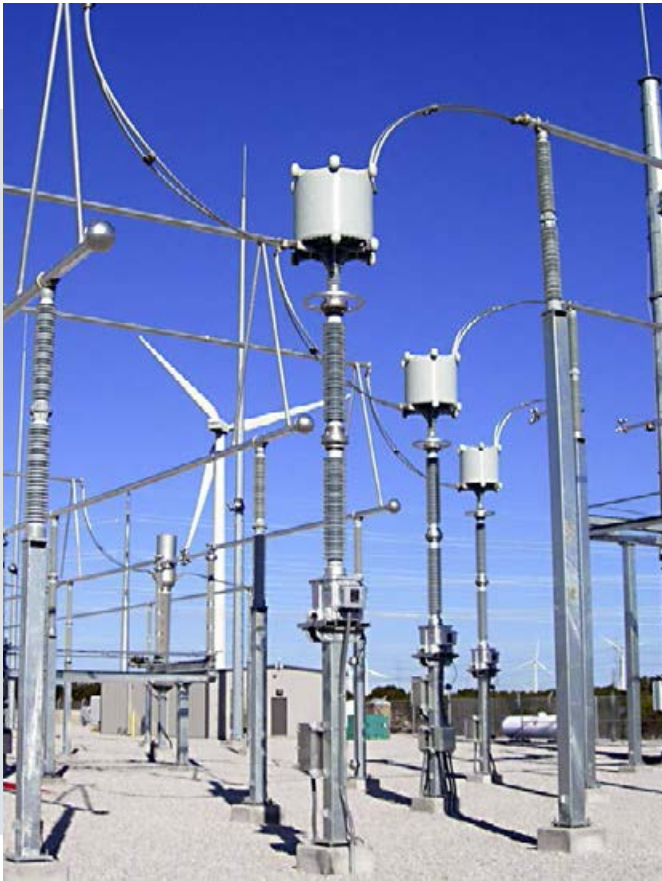
Fig. 65: Line traps
