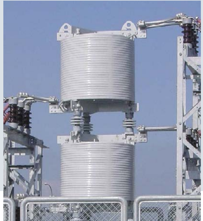
Fig. 66: 3-phase stacked current-limiting reactor
