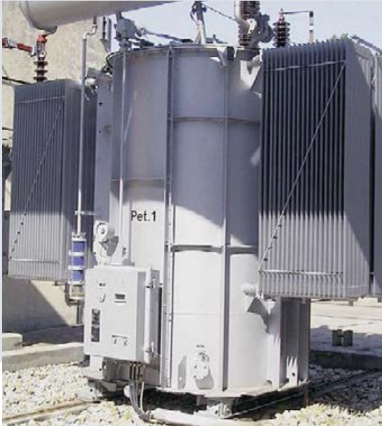
Fig. 69: Arc-suppression coil 110 kV
