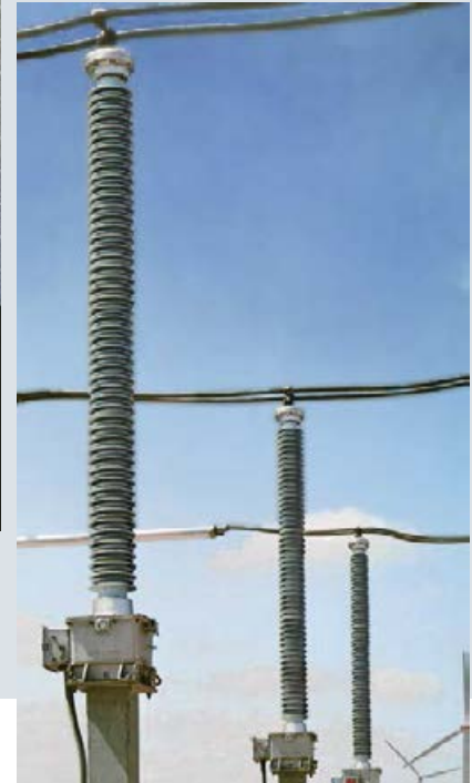
Fig. 52: 245 kV capacitor voltage transformers at Oncor substation (USA)
