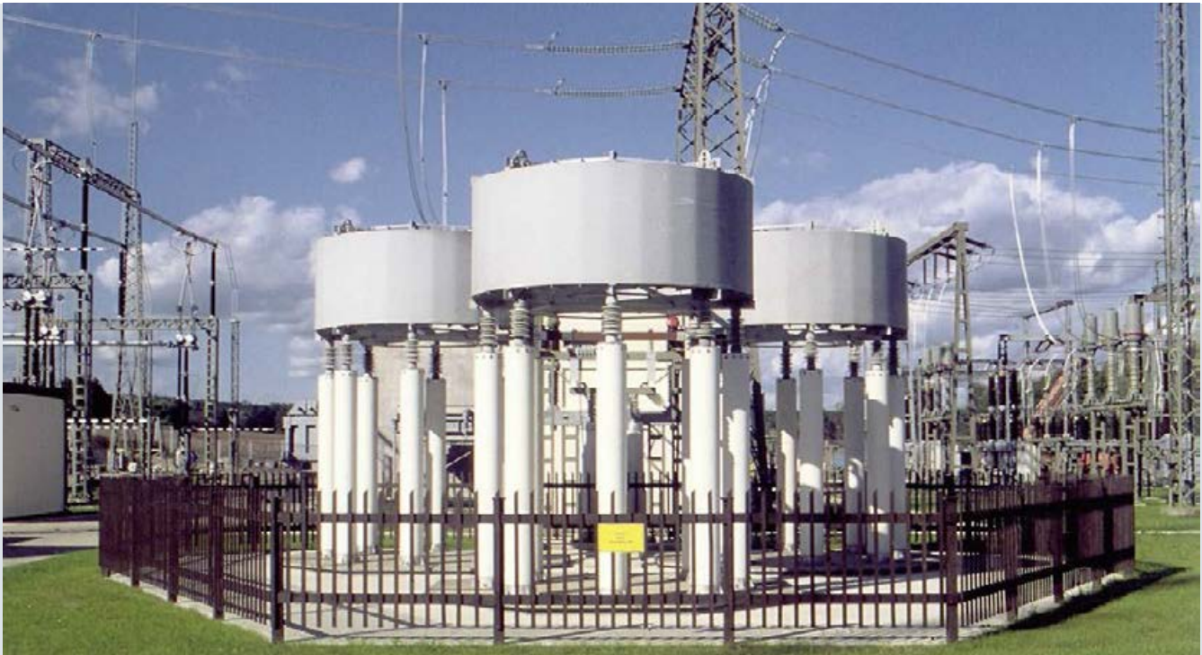
Fig. 67: Tertiary-connected shunt reactors
