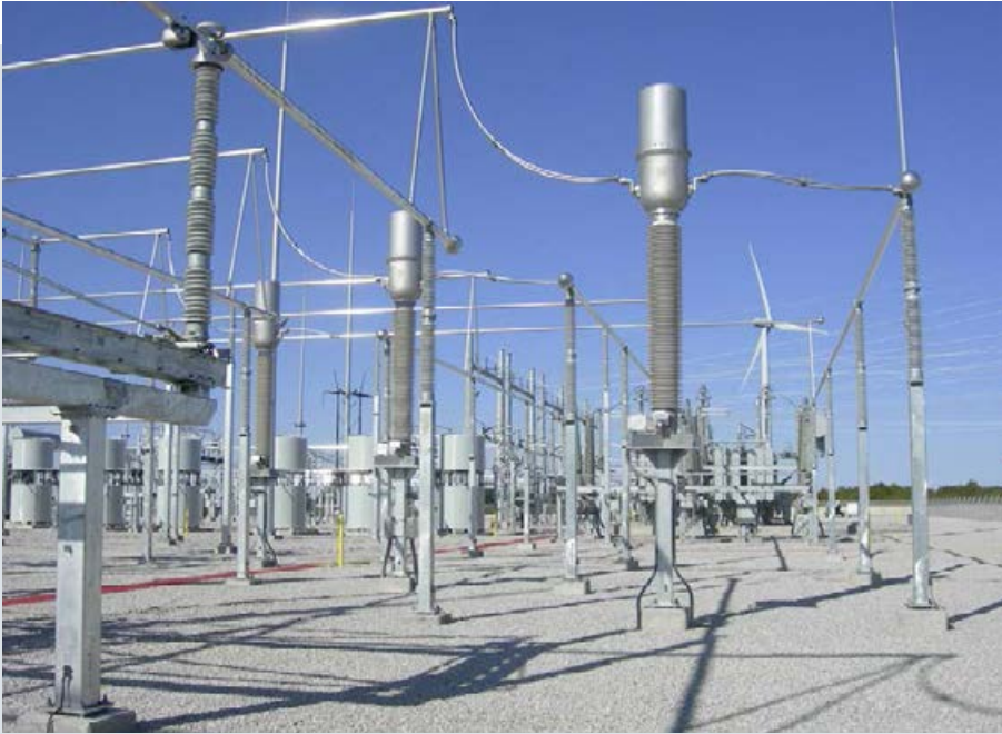
Fig. 53: 362 kV gas-filled combined instrument transformer
