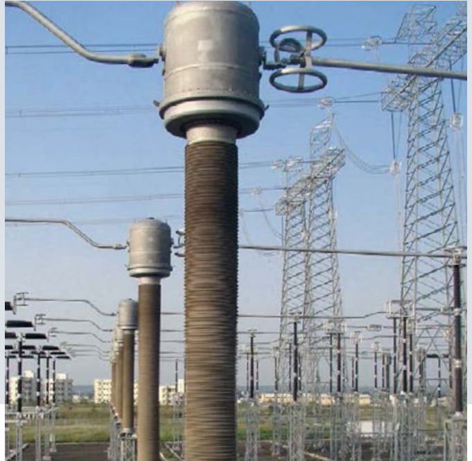
Fig. 45: 800 kV gas-insulated current transformers
