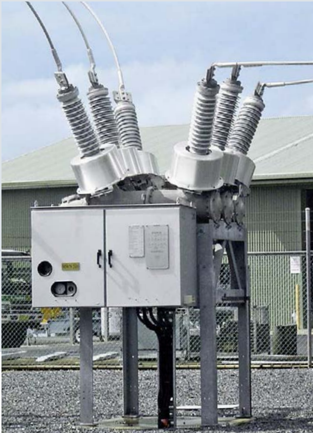
Fig. 11: SPS2/3AP1 DT 72.5 kV
