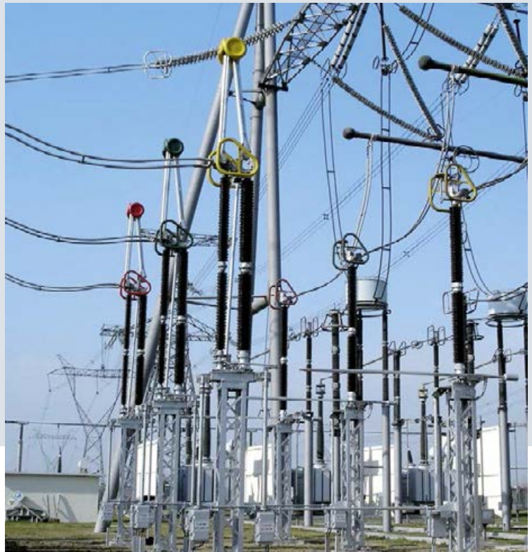
Fig. 29: Knee-type disconnector
