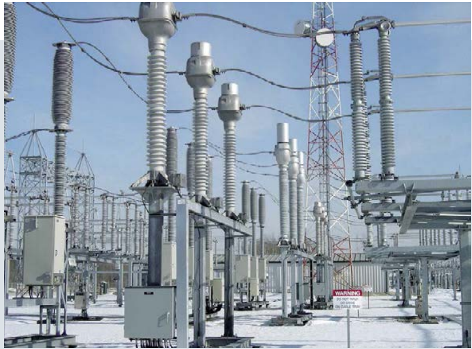
Fig. 47: 300 kV oil-immersed current transformers in Alberta, Canada
