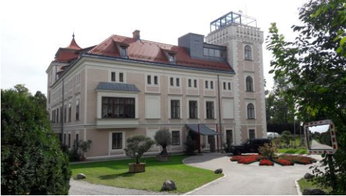
SCHLOSS LEOPOLDSDORF Castle, Office Building
