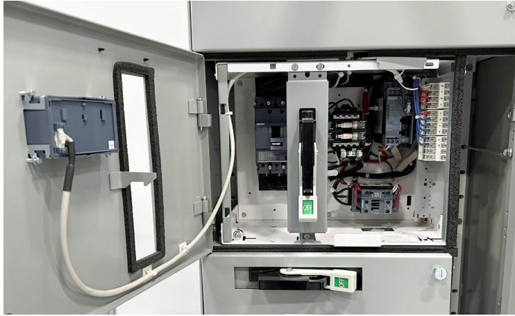
Example of Full Voltage Non-Reversing (FVNR)
