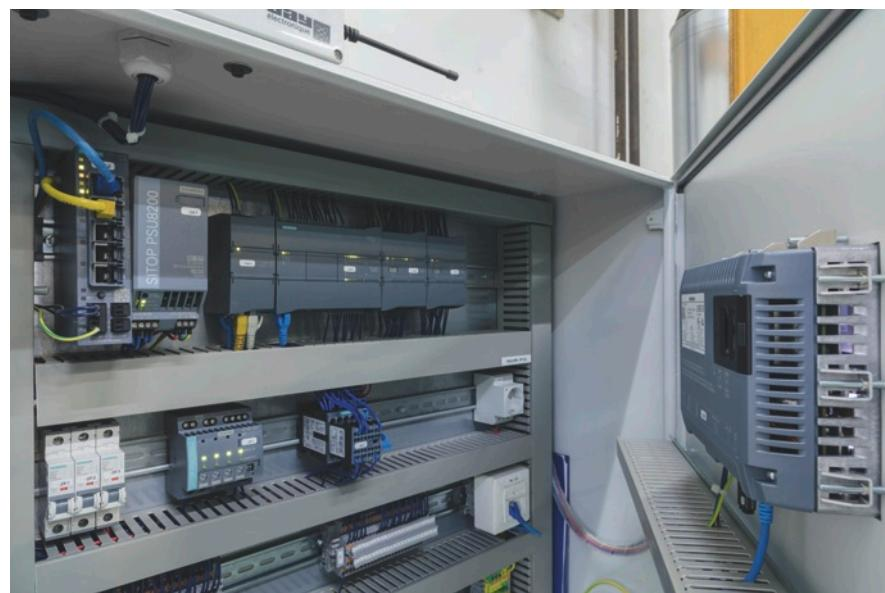
Various Siemens devices in the control cabinet: Also installed besides the SCALANCE S615 security modules are the SITOP PSE200U selectivity and diagnostic module as well as the SITOP PSU8200 24 V DC power supplies.
