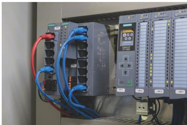
Compact automation technology optimally integrated in the control cabinet: The SCALANCE S615 security module together with the SCALANCE XC108 Industrial Ethernet managed switch and the SIMATIC S7-1500 controller.
