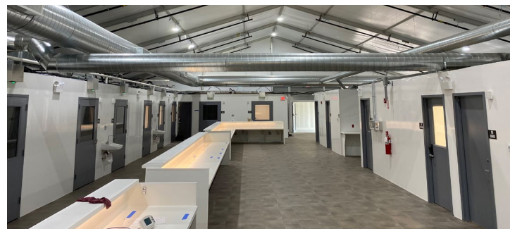
Interior of a modular healthcare facility in White Plains, NY, where Siemens supplied critical infrastructure technologies.
