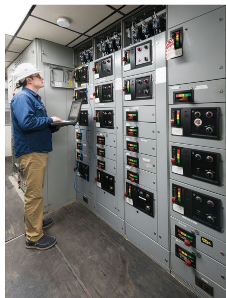
Tony DeSalvo, global automation and controls support supervisor, takes readings from a drilling rig motor control center recently upgraded with Siemens SIMOCODE motor management system.
