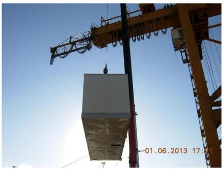
Replace the whole E-Room as fully containerized solution Scope:
