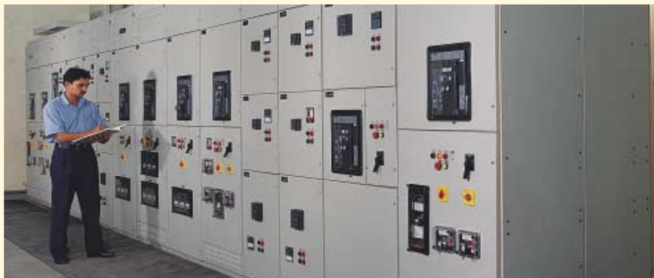
Siemens Low Voltage Switchboards installed at Baan IT Park at Hyderabad.
