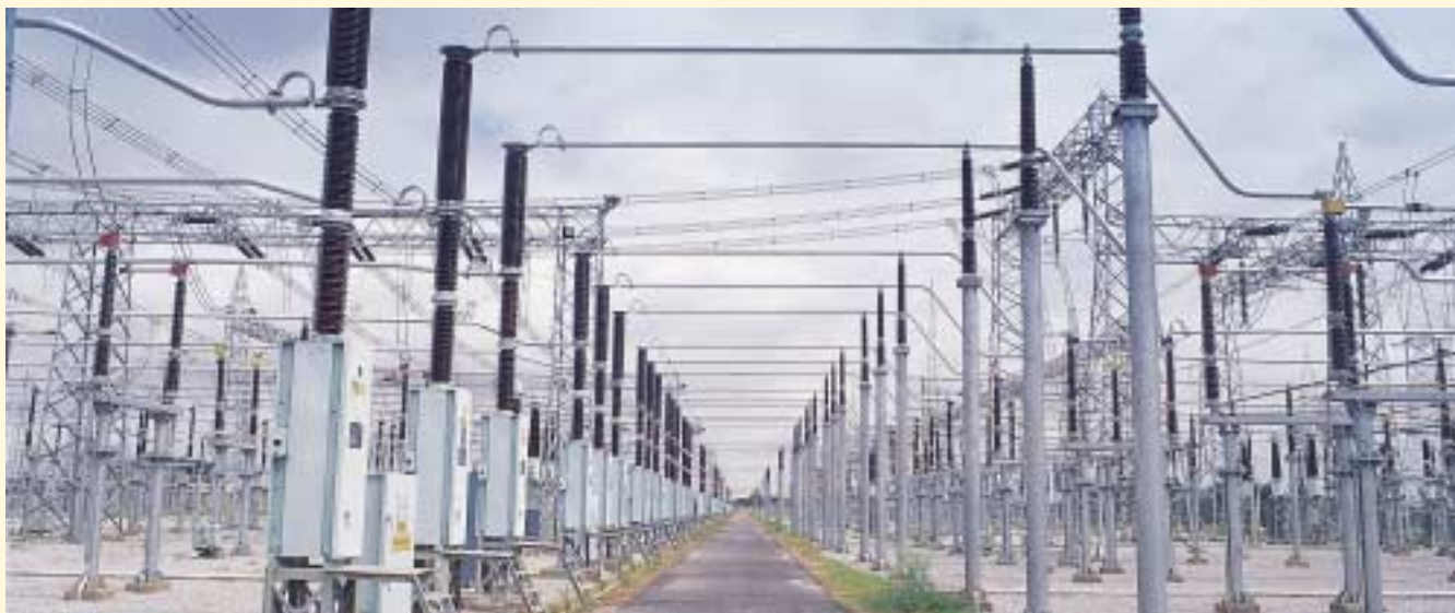
Installation of 220 kV breakers for KPTCL at Neelamangala, Karnataka.
