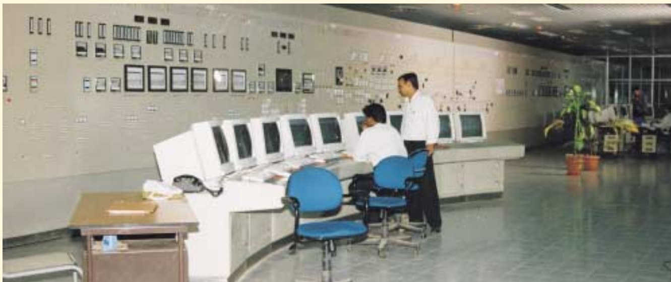
Power Plant Automation Systems installed at Gujarat Industries Power Company Ltd. - Surat Lignite Power Project.
