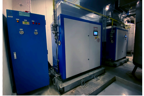
Temperature sensors control the speed and operation of the fan to prevent system failures from overheating and maintain room ventilation.
