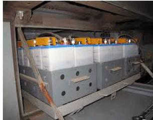
Figure 4-2: Typical Crossing Battery Banks
