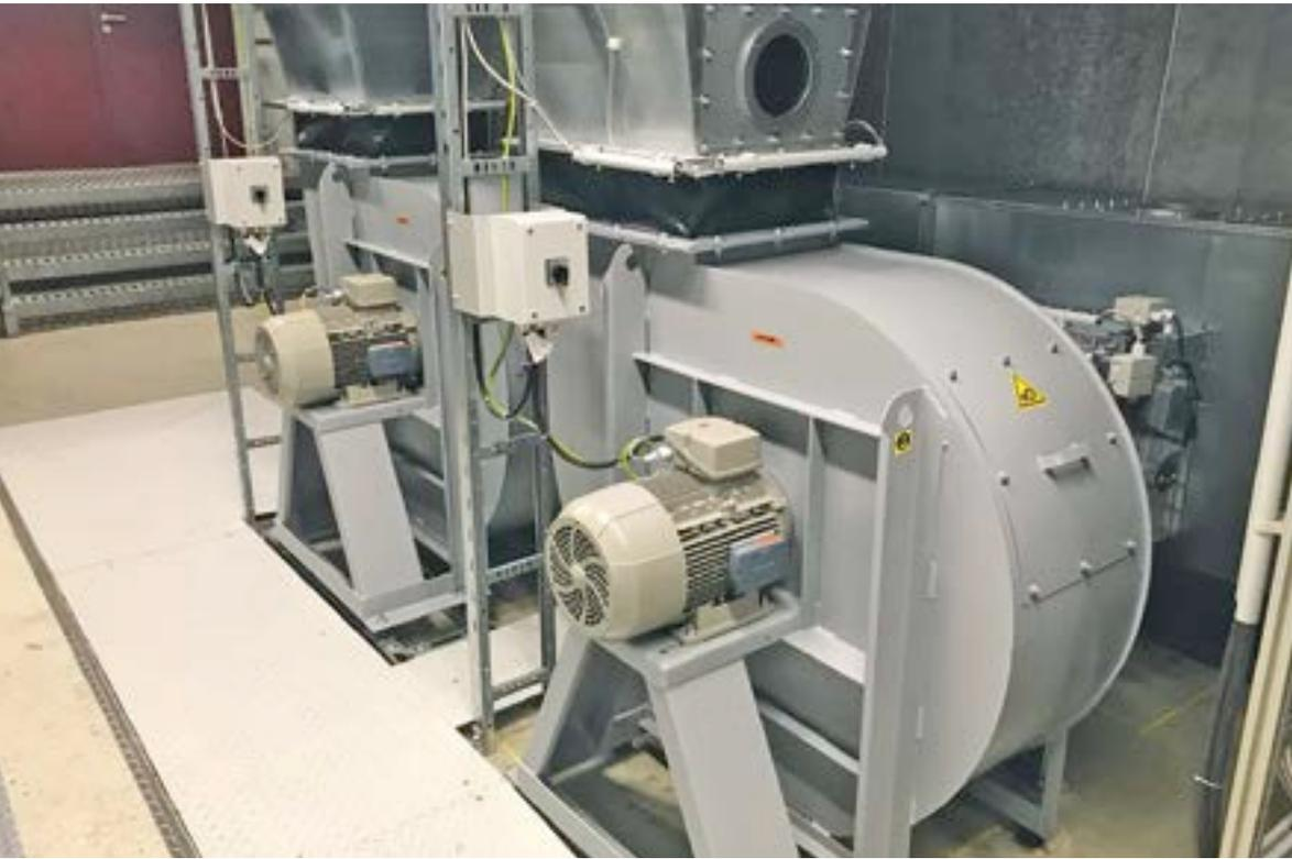
Fig. Process air extraction system for GWE production areas
