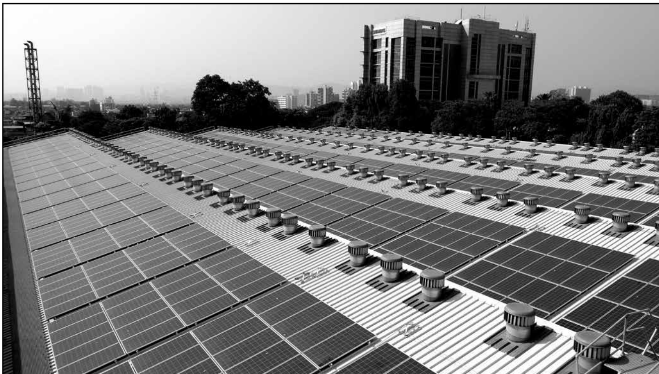
Roof-top solar panels spread over a total area of 12,500 square meters installed in Kalwa - almost equivalent to the area of two soccer fields
