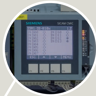
SICAM CMIC installed in a separate RTU cubicle inside the transformer substation
