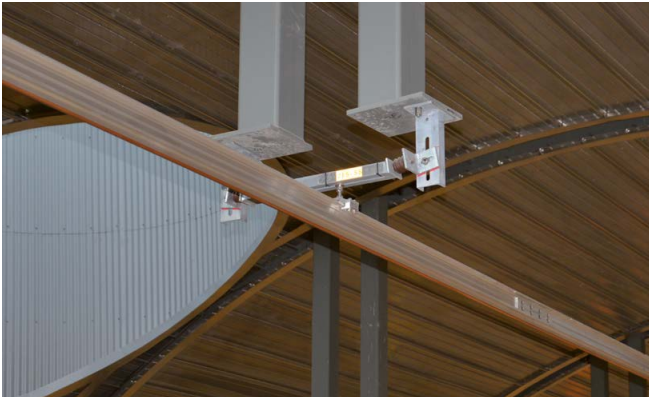
Deckenstromschiene, Westbrook Station Calgary, Kanada
