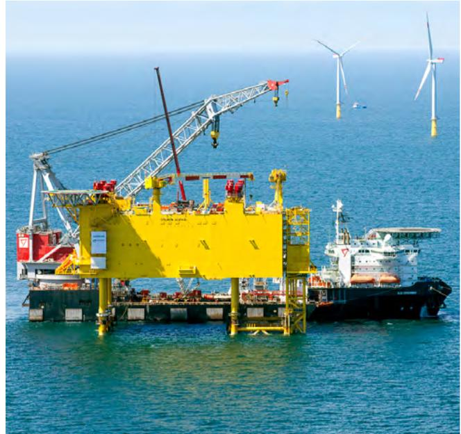
Fig. 2.2-37: SylWin 1, 864 MW HVDC PLUS, North Sea
