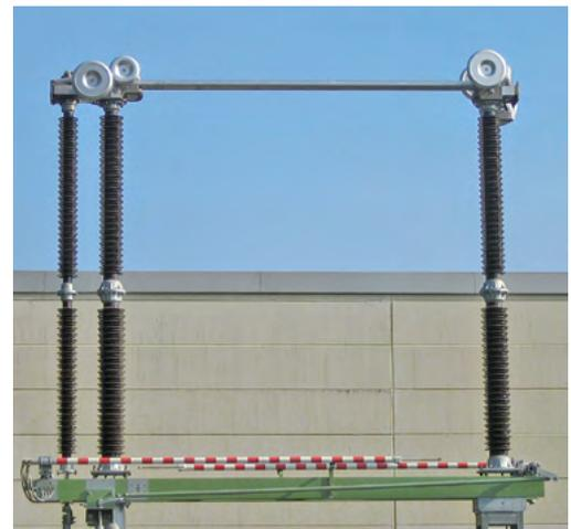
Fig. 4.1-27: Vertical-break disconnector
