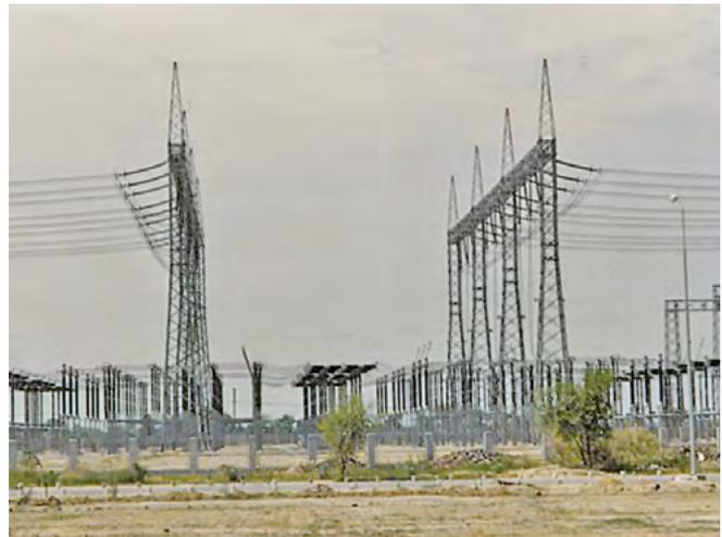
Fig. 3.1-20: One-breaker-and-a-half arrangement, 500 kV, Pakistan
