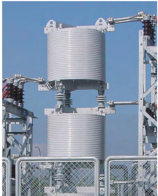
Fig. 4.2-34: 3-phase stacked current-limiting reactor
