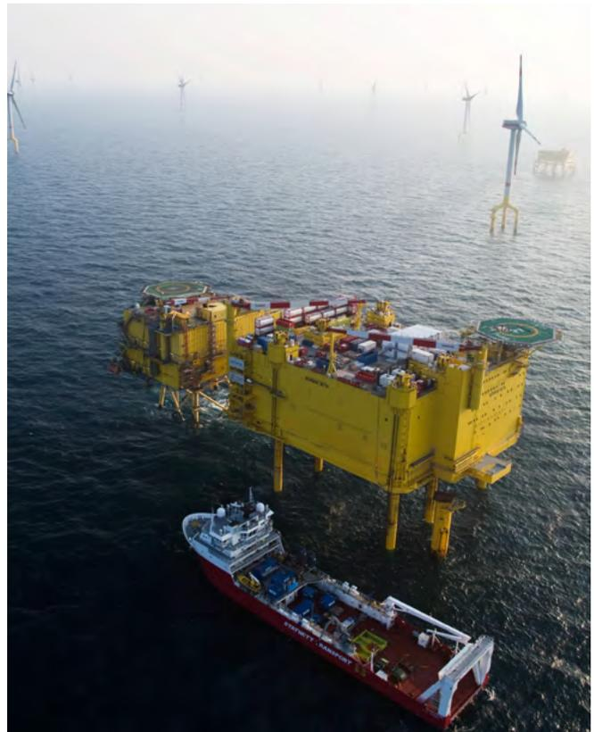
Fig. 2.2-35: BorWin 2, 800 MW HVDC PLUS, North Sea
