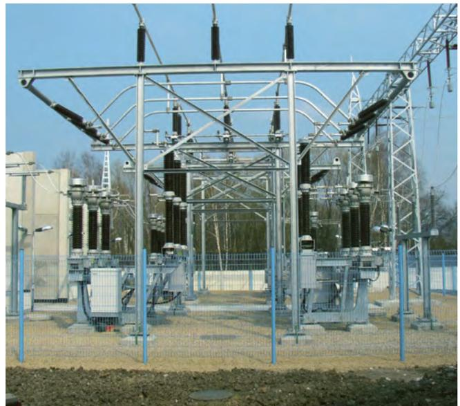
Fig. 3.1-26: H-arrangement with SIMOVER, 145 kV, Czech Republic
