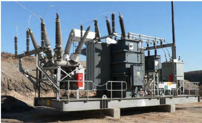
Fig. 2.4-14: 145kV 10MVA skid substation
