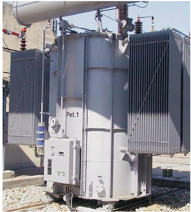
Fig. 4.2-37: Arc-suppression coil 110 kV
