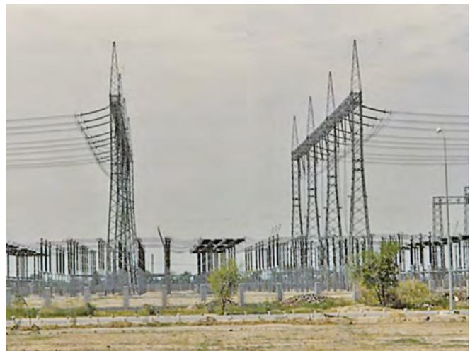
Fig. 3.1-20: One-breaker-and-a-half arrangement, 500 kV, Pakistan
