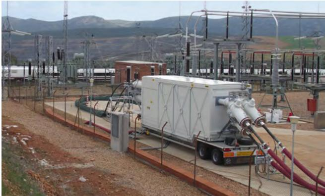
Fig. 2.4-13: 245kV Mobile substations with HV cable connection
