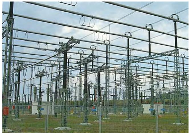
Fig. 3.1-18: Busbar disconnectors in diagonal arrangement, 380 kV, Germany
