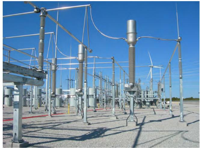
Fig. 4.2-21: 362 kV gas-filled combined instrument transformer
