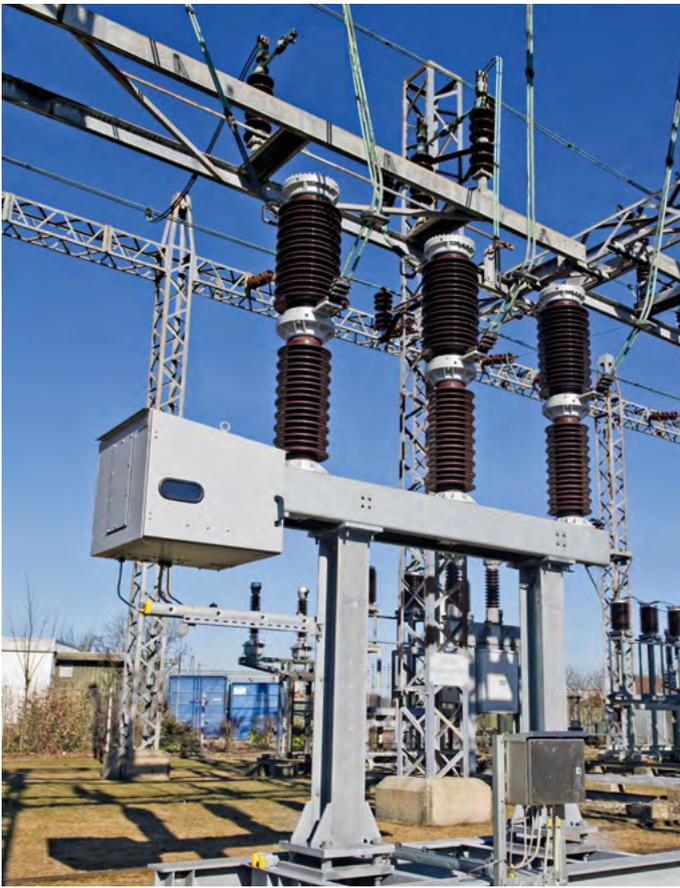
Fig. 4.1-10: 3AV1 FG vacuum circuit-breaker 72.5 kV
