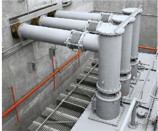
Fig. 3.1-46: Transformer termination
