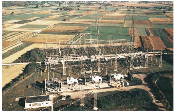
Fig. 3.1-2: Air-insulated outdoor switchgear
