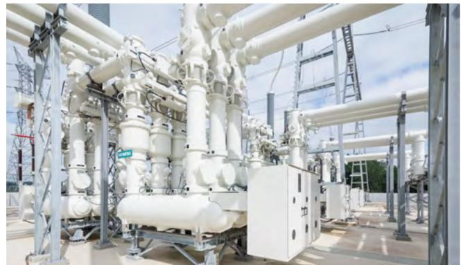
Fig. 3.1-40: 8DQ1 switchgear for a rated voltage of 420 kV
