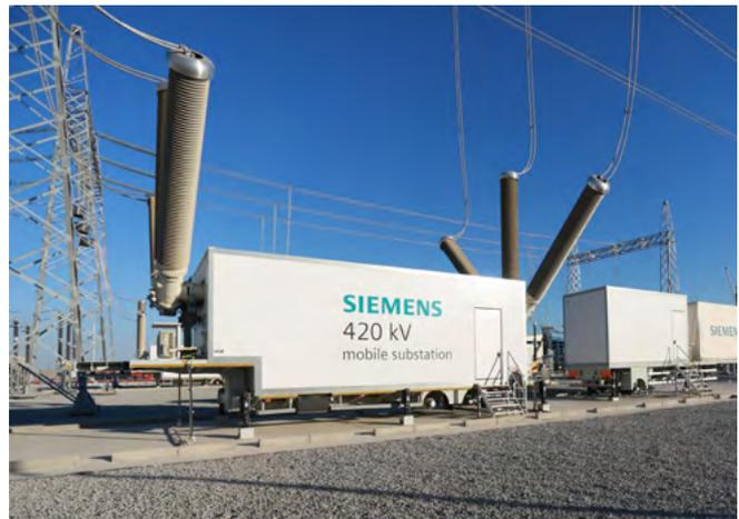
Fig. 2.4-24: world first 420kV mobile substation
