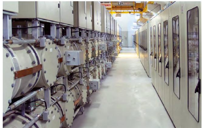
Fig. 3.1-35: 8DN8 GIS for a rated voltage of 145 kV
