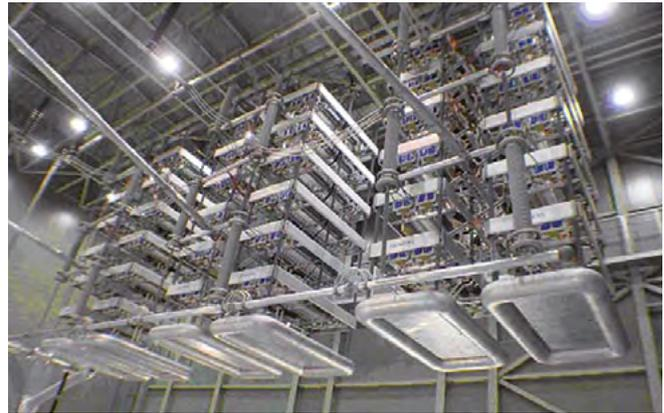
Fig. 2.2-2: Earthquake-proof and fire-retardant thyristor valves in 500 kV long-distance transmission in Guizho-Guangdong, China
