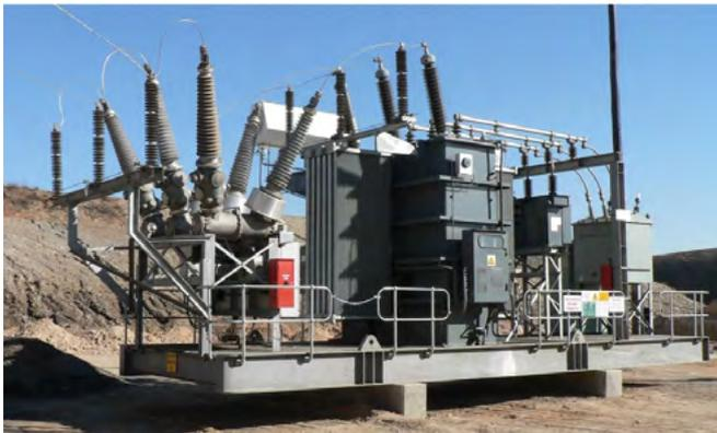
Fig. 2.4-14: 145kV 10MVA skid substation
