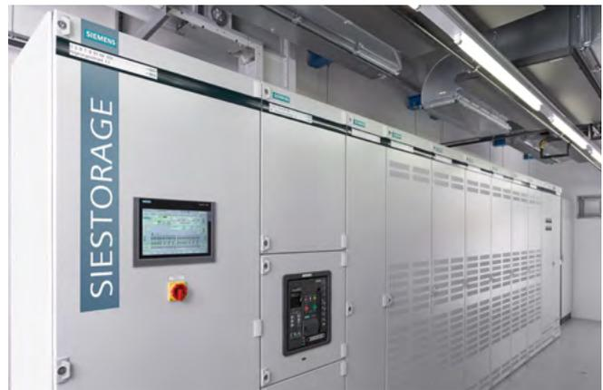
Fig. 2.3-16: SIESTORAGE system installed in an existing electrical building at the steel mill of the AMEH in Eisenhüttenstadt, Germany
