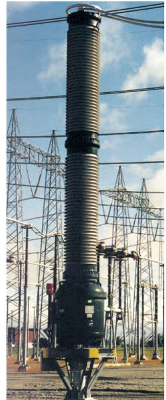
Fig. 4.2-14: 800 kV gas-insulated current transformers
