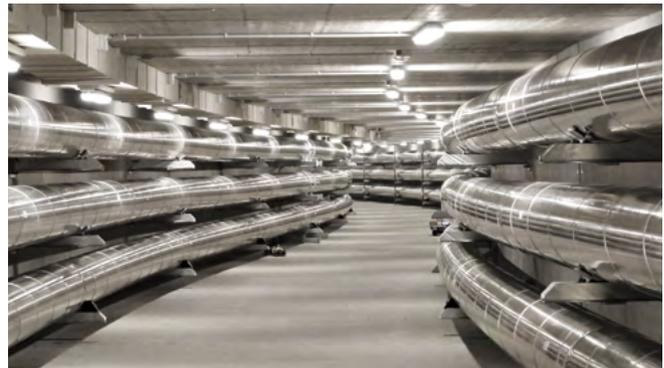
Fig. 2.2-46: GIL tunnel installation, Munich, Germany
