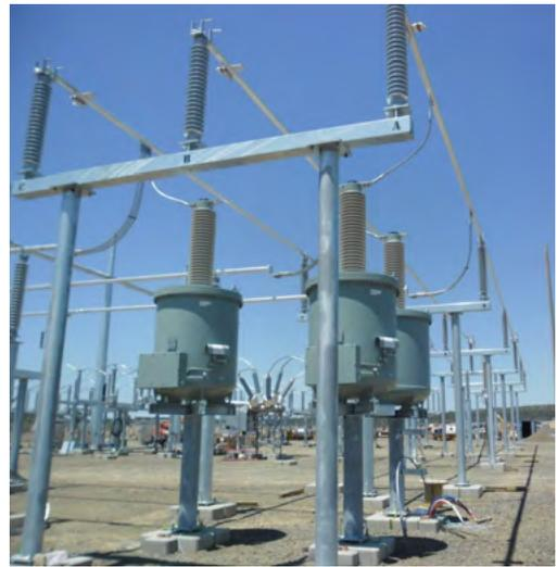
Fig. 4.2-29: 145 kV power VT for AIS
