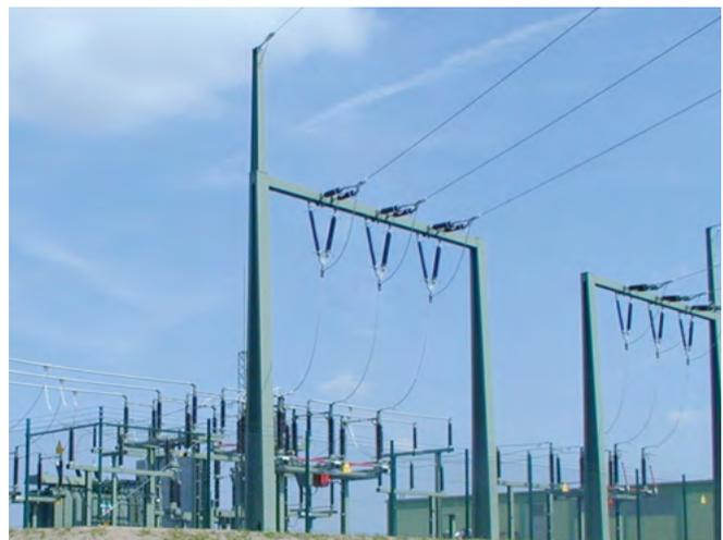
Fig. 3.1-12: H-arrangement, 110 kV, Germany
