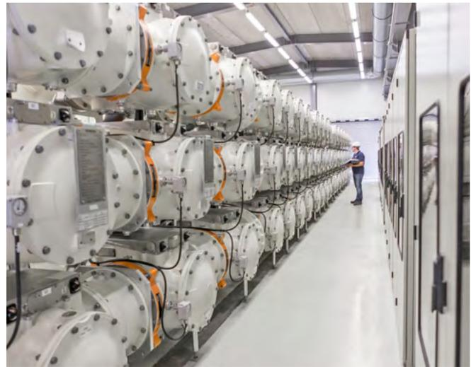
Fig. 3.1-31: 8DN8 GIS for a rated voltage of 110 kV
