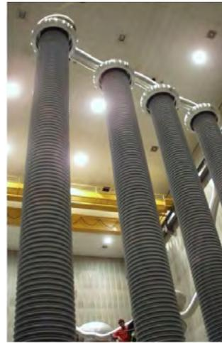
Fig. 4.2-22: Energy storage capacitor
