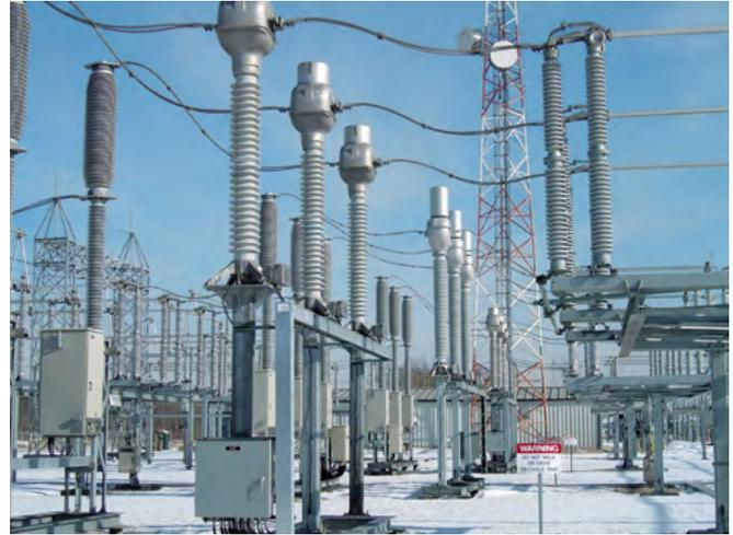
Fig. 4.2-15: 300 kV oil-immersed current transformers in Alberta, Canada
