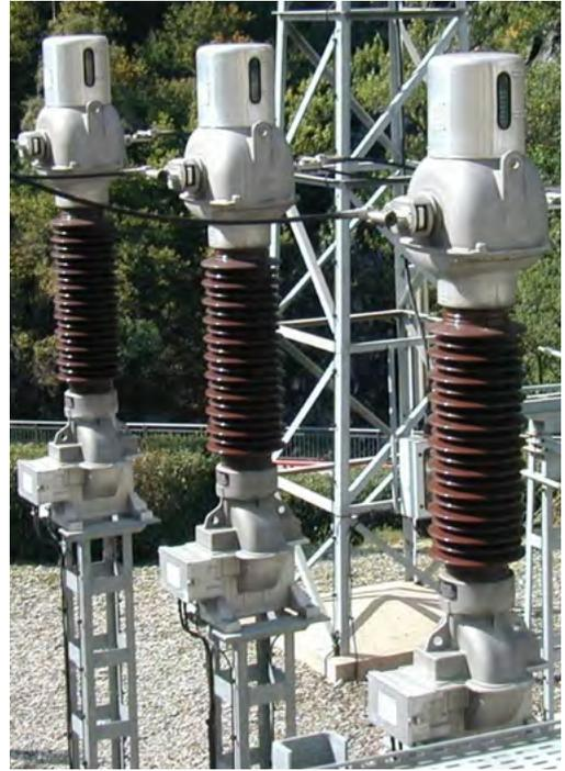
Fig. 4.2-18: 145 kV oil-immersed combined instrument transformer
