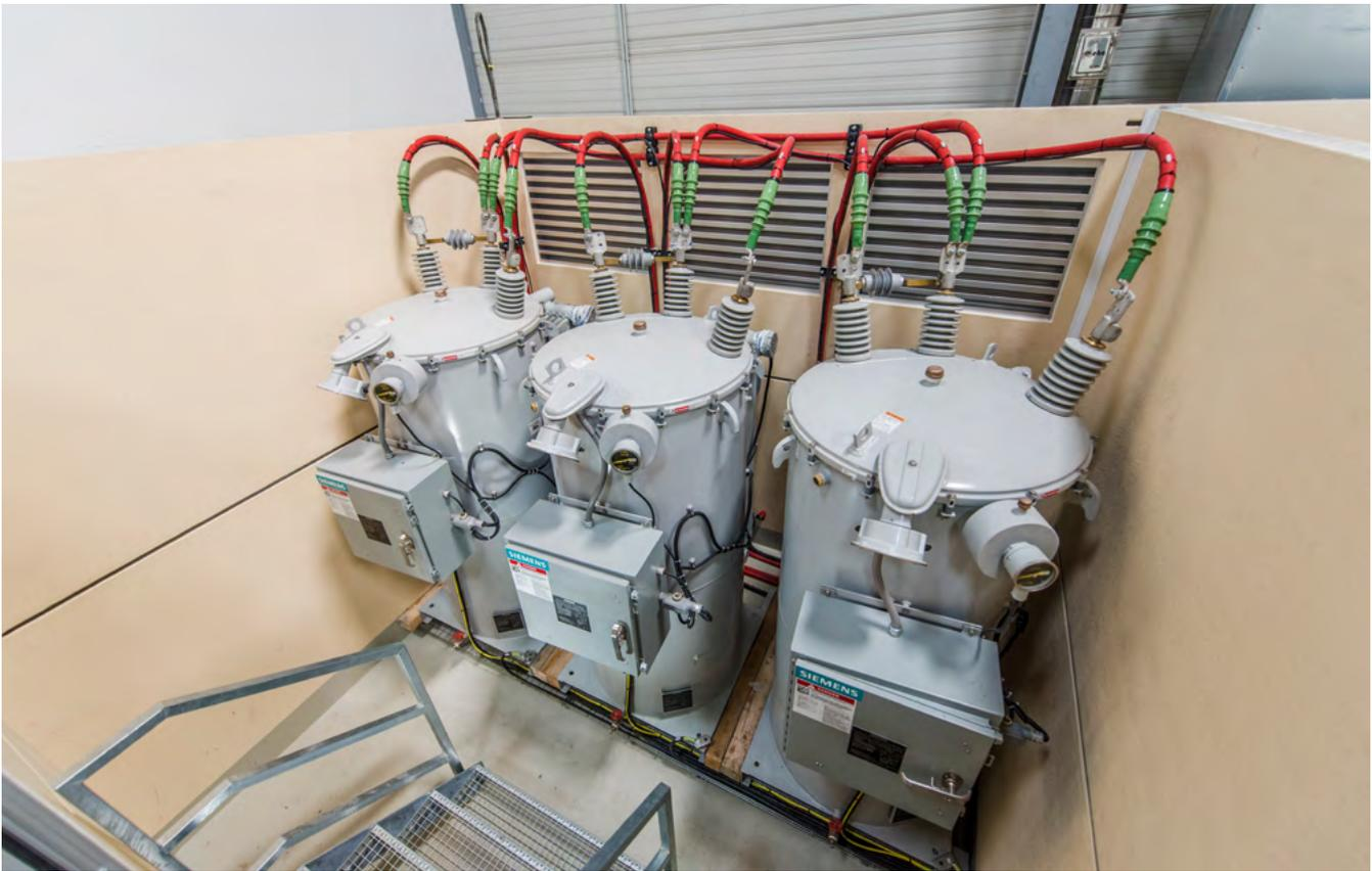
Fig. 5.11-4: In-phase voltage regulators, Niederstetten, Germany
