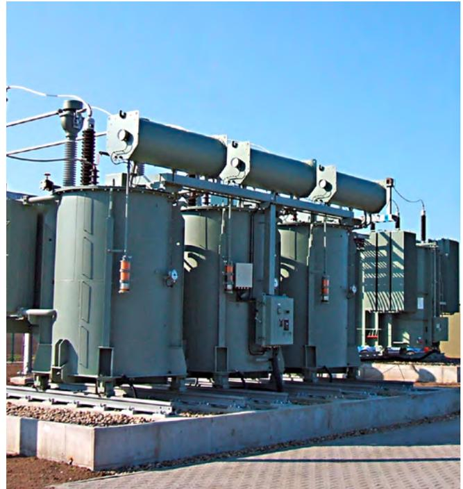
Fig. 4.2-38: Variable shunt reactor
