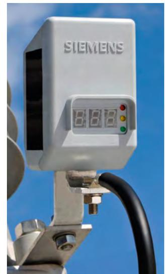
Fig. 4.2-11: Arrester condition monitor (ACM)
