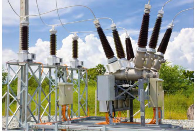
Fig 3.1-27: Dead Tank Compact (DTC)
