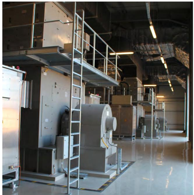
Fig. 2.2-26: Synchronous condenser building of the HVDC Black Sea Transmission Network, Georgia
