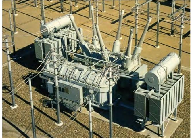
Fig. 5.9-1: Phase-shifting transformer
