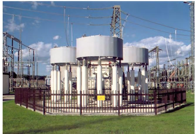
Fig. 4.2-35: Tertiary-connected shunt reactors
