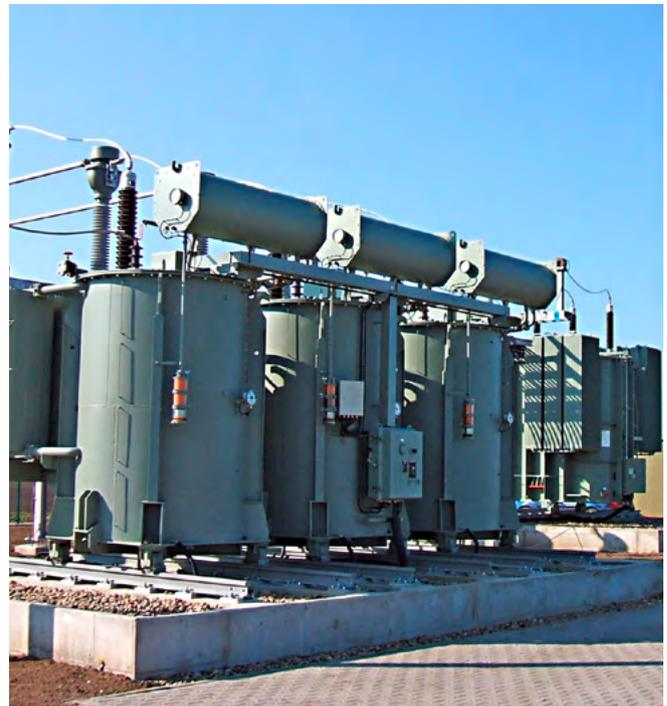
Fig. 4.2-38: Variable shunt reactor
