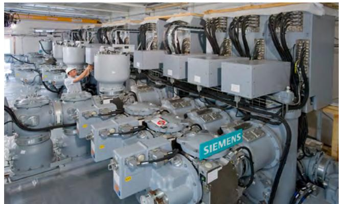
Fig. 2.4-3: High Voltage GIS E-house project for a mine, New Caledonia
