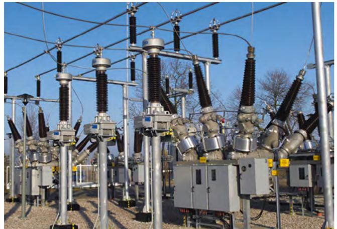
Fig. 4.1-17: 3AP1 DTC 145 kV
