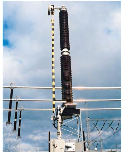
Fig. 4.1-30: Free-standing earthing switch
