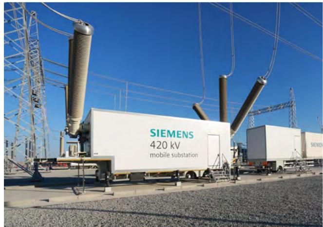
Fig. 2.4-24: world first 420kV mobile substation
