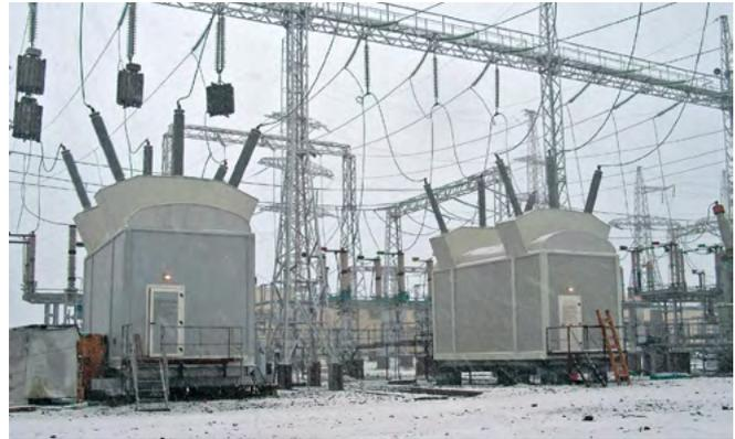
Fig. 2.4-7: 245kV E-house for Transmission utility in Siberia
