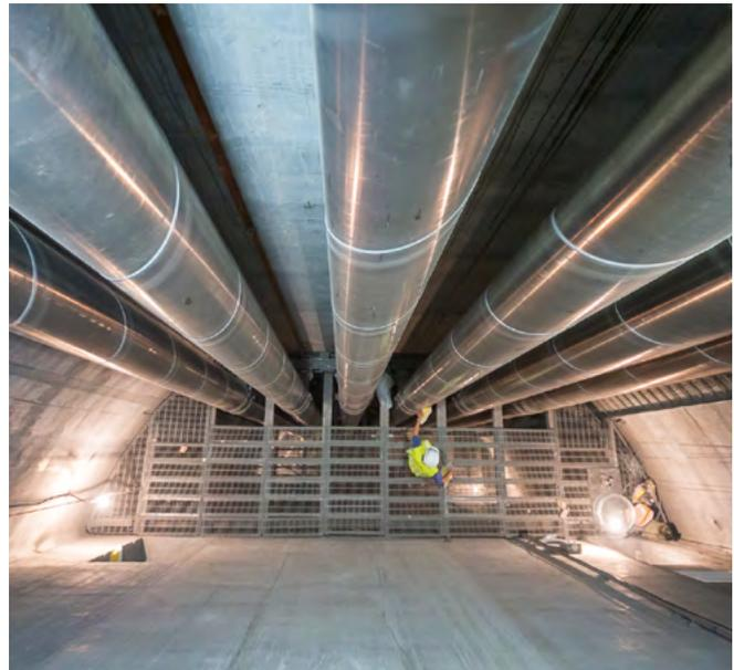
Fig. 2.2-51: Vertically installed GIL in Xiluodu, China
