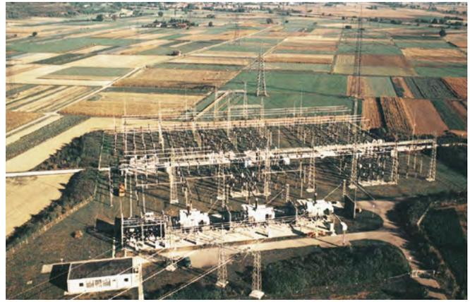
Fig. 3.1-2: Air-insulated outdoor switchgear
