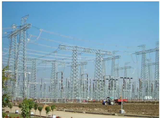
Fig. 3.1-22: One-breaker-and-a-half arrangement, 800 kV, India
