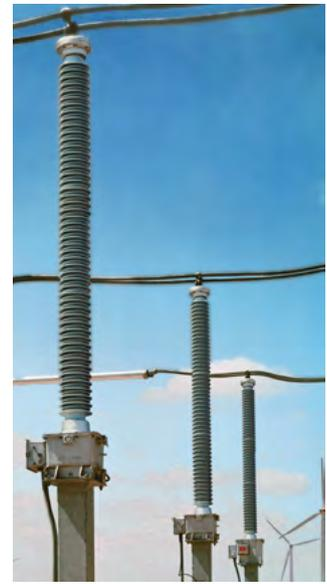
Fig. 4.2-20: 245 kV capacitor voltage transformers at Oncor substation (USA)
