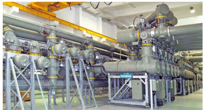
Fig. 3.1-39: 8DQ1 switchgear for a rated voltage of 550 kV
