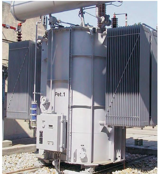
Fig. 4.2-37: Arc-suppression coil 110 kV
