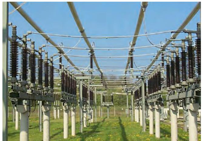
Fig. 3.1-14: Busbar disconnectors "in line", 110 kV, Germany
