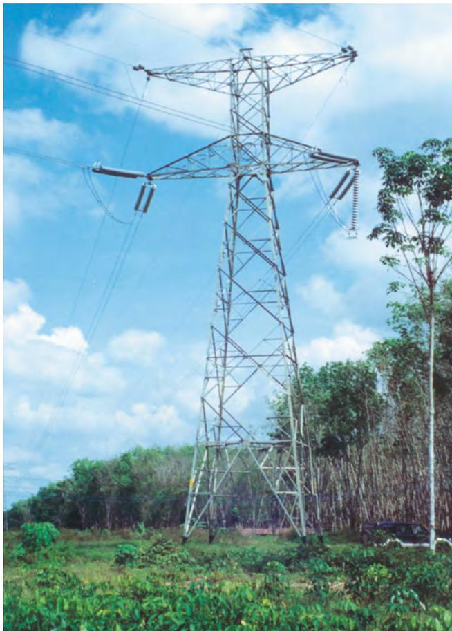
Fig. 2.2-76: 300 kV HVDC interconnector from Thailand to Malaysia (bipole transmission line)
