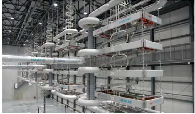
Fig. 2.2-5: UH voltage and power electronics – the thyristor valves are designed to operate at 800 kV voltage level. Yunnan-Guangdong, China
