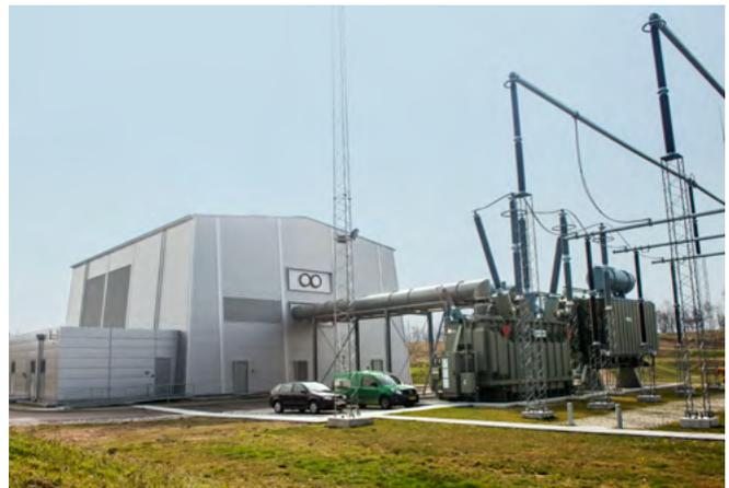
Fig. 2.2-25: Synchronous condenser in Bjaeverskov, Denmark
