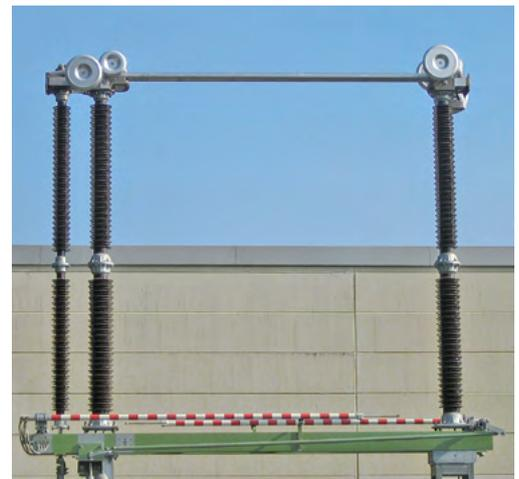
Fig. 4.1-27: Vertical-break disconnector
