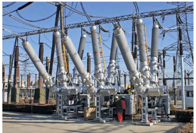
Fig. 4.1-18: 3AP1 DTC 245 kV
