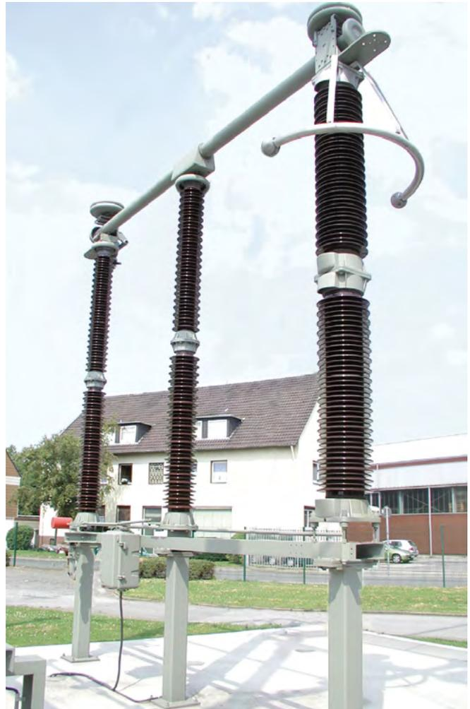
Fig. 4.1-28: Double-side break disconnector with integrated surge arrester
