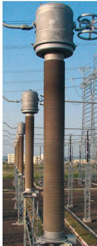
Fig. 4.2-13: 420 kV gas-insulated current transformers
