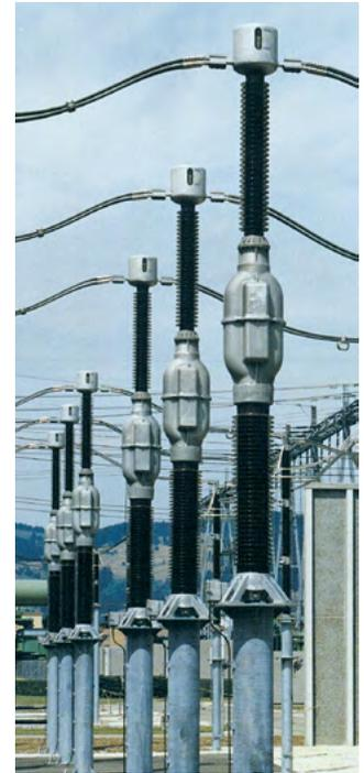
Fig. 4.2-17: 420 kV oil-paper-insulated inductive voltage transformers
