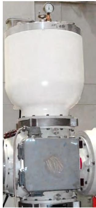
Fig. 4.2-27: 145 kV inductive voltage transformer for GIS
