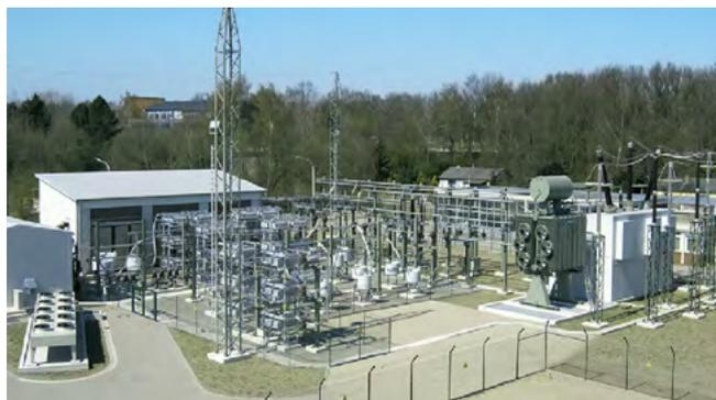
Fig. 2.2-19: Static Var Compensator (SVC) installation
