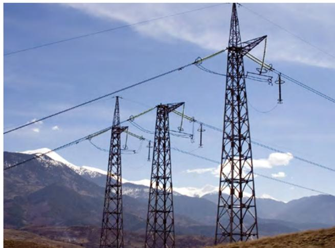
Fig. 4.2-3: 400 kV line in Bulgaria, NGLA solution realized with 3EL2
