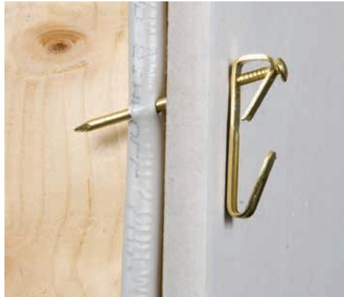
Example of line-to-ground arc fault (nail puncturing NM-B wire)
