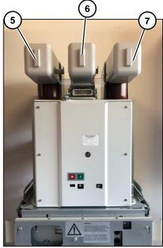
Fig. 144: Circuit breaker / fuse combination on the service truck
