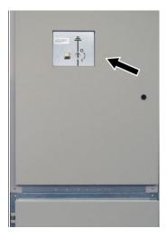
Fig. 235: Control elements of earthing switch for busbar system
