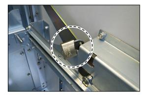
Fig. 249: Padlocking the shutter mechanism on the right side in the switching-device compartment
