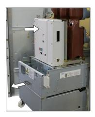
Fig. 115: Pushing the withdrawable circuit-breaker into the panel
