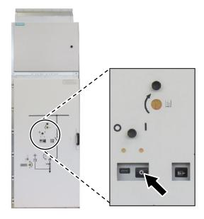
Fig. 65: Position indicator on the circuit-breaker, OPEN
