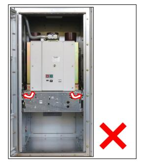
Fig. 94: Circuit-breaker panel without service truck
