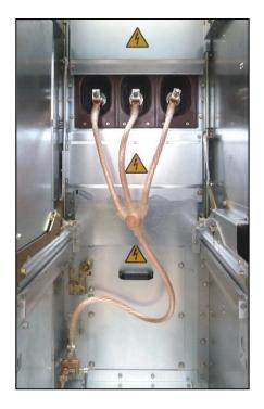
Fig. 339: Earthing device completely mounted
