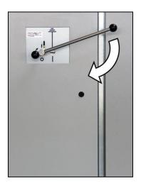
Fig. 230: Closing the busbar earthing switch
