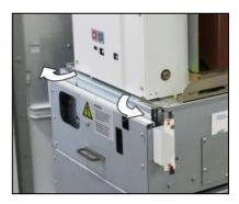
Fig. 113: Releasing the interlocking of the withdrawable circuit-breaker
