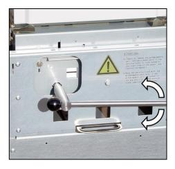
Fig. 109: Operating the feeder earthing switch operating shaft
