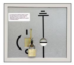
Fig. 247: Operating slide on busbar earthing switch padlocked
