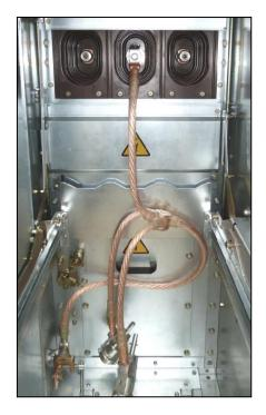
Fig. 338: Earthing tulip fixed on central bushing contact
