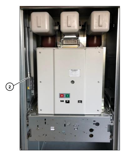
Fig. 141: Low-voltage connector placed on the side wall
