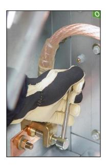
Fig. 347: Unscrewing the earthing clamp
