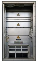
Fig. 285: Ventilation duct placed centrally on the panel base frame
