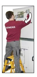
Fig. 231: Closing the busbar earthing switch using an electrician's ladder
