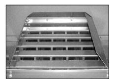
Fig. 397: View from above onto a ventilation unit in the pressure relief duct
