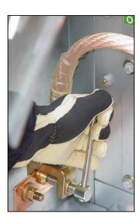
Fig. 331: Bolting the earthing clamp
