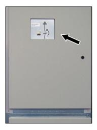
Fig. 222: Control elements of earthing switch for busbar system
