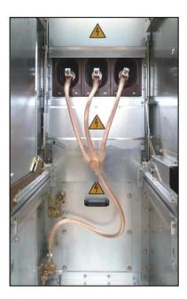
Fig. 340: Earthing device to be removed
