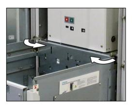
Fig. 118: Interlocking the withdrawable circuit-breaker
