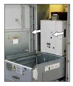
Fig. 99: Pulling out the withdrawable circuit-breaker, type 3AE5
