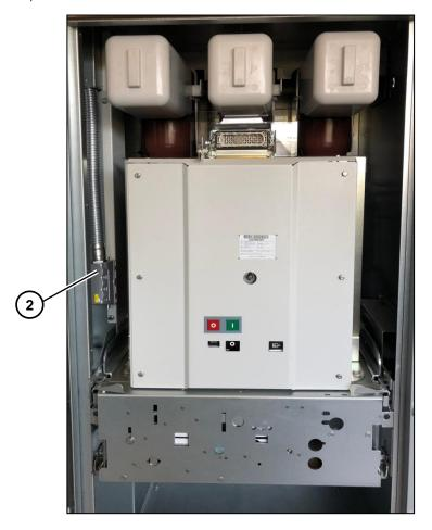
Fig. 139: Low-voltage connector placed on the left side
