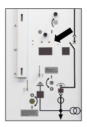
Fig. 382: Circuit-breaker type 3AE5: actuating opening for closing the circuit-breaker manually
