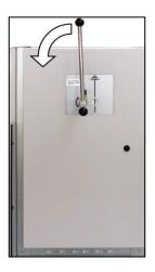
Fig. 243: Opening the busbar earthing switch
