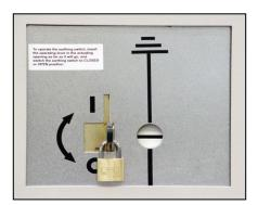
Fig. 225: Operating slide on busbar earthing switch padlocked
