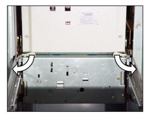
Fig. 98: Unlocking the withdrawable circuit-breaker
