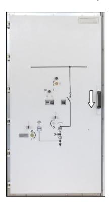
Fig. 36: Closing the high-voltage door of the circuit-breaker panel
