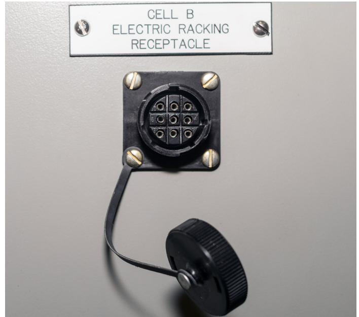
Figure 6: Connector for control pendant cable connection
