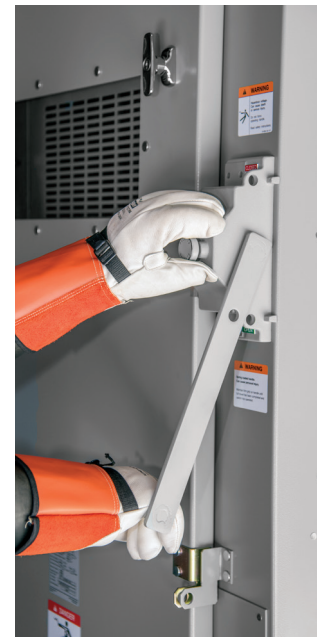
Figure 61: Operation of the load-interrupter switch
