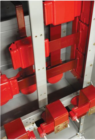
Figure 20: Main bus with insulating boots installed (bus compartment covers removed)
