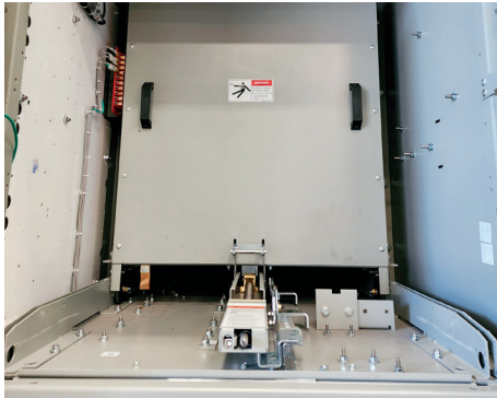
A. VT rollout tray in CONNECTED position. Handle/interlock bar fully extended to secure VT rollout tray in cell.
