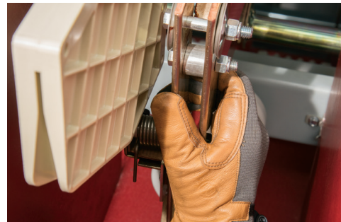
Figure 64: Disengage switch blades
