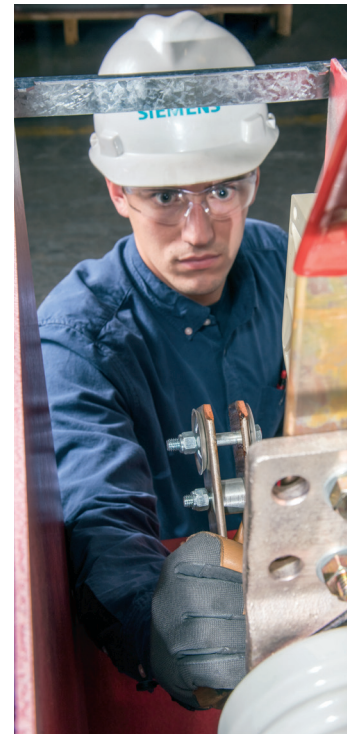
Figure 66: Reconnect pushrods
