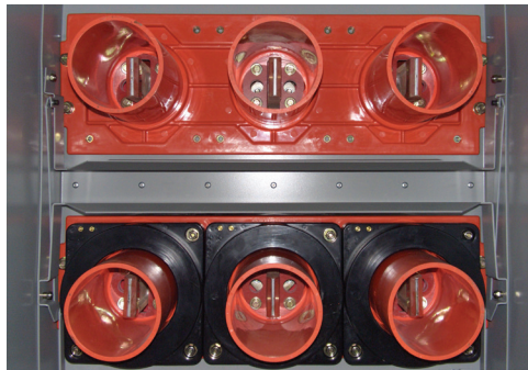
Figure 36: Type MD current transformers installed on lower disconnects (barrier removed for photo)
