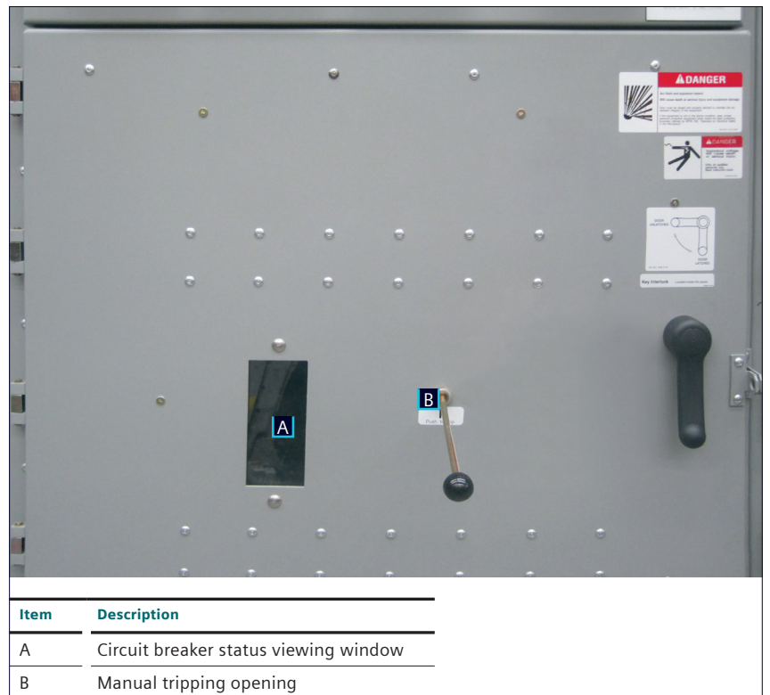
Figure 41: Manual tripping of circuit breaker
