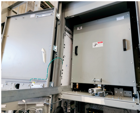
C. Extension rail being inserted.
