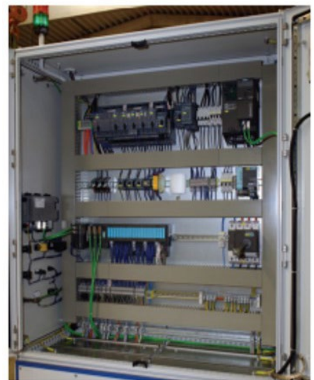
Space savings in the control cabinet. The SIRIUS 3RA6 compact starters and the SIMATIC ET200SP distributed controller support transparent electrical engineering and easy communication via PROFINET.
