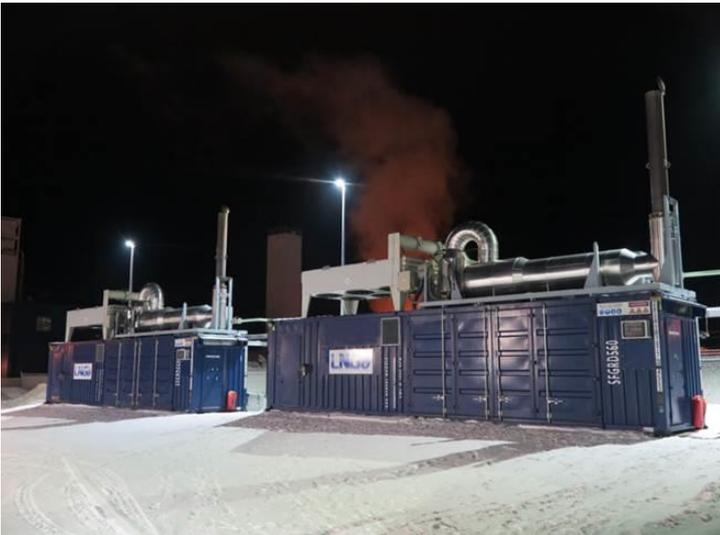
**(Above): Siemens' lean-burn gas engines provide power to the LNGo HP process.**
