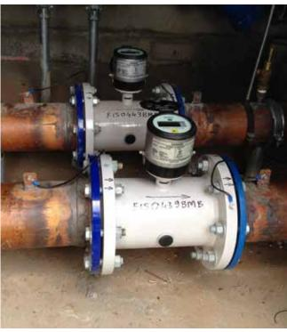
City West Water has installed more than 1000 SITRANS F M MAG 8000 meters throughout Melbourne.
