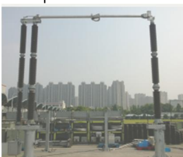
Knee-type disconnector 3DN5 in closed position
