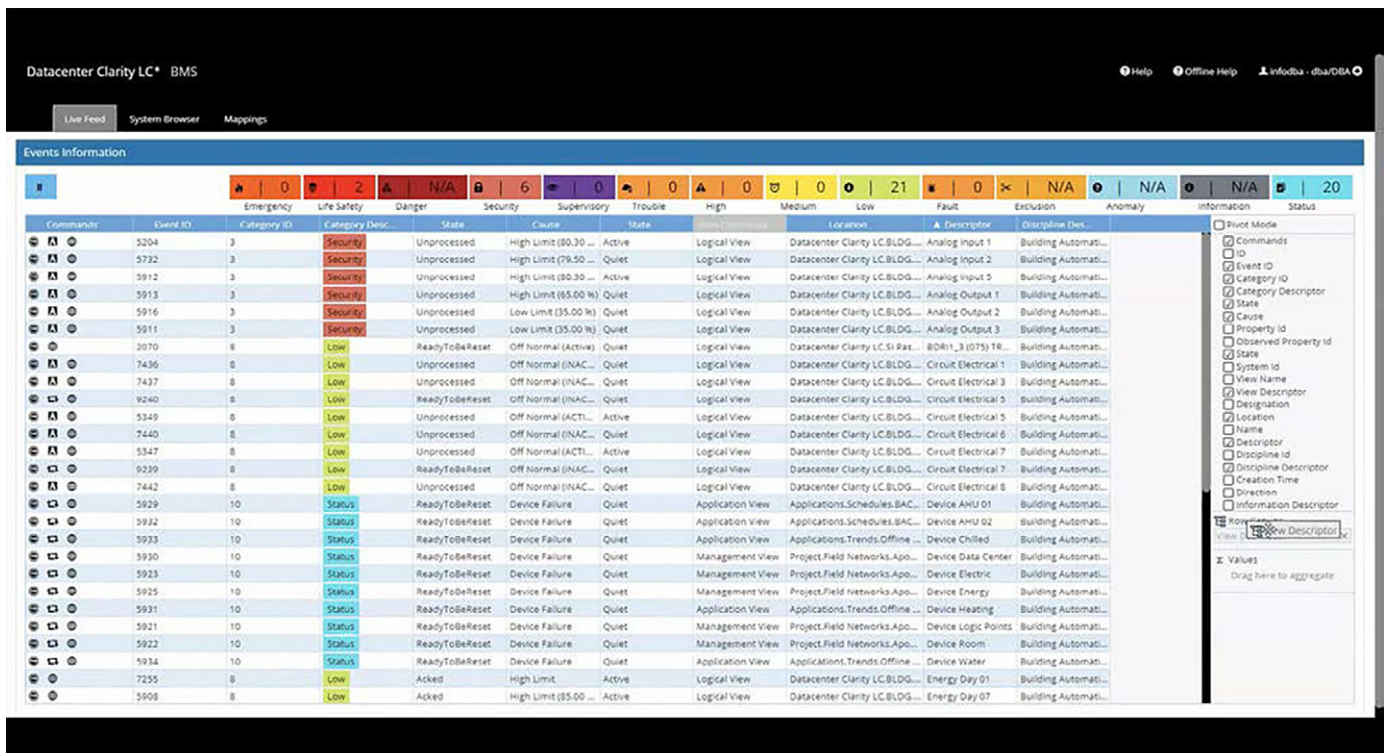
Datacenter Clarity LC view of the Desigo CC alarms
