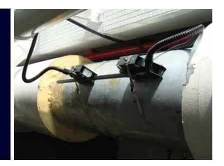
mance records of Siemens clamp-on energy meters in similar applications at other universities, and what they discovered was that several dozen elite universities throughout the United States have been using these meters for years to optimize chiller load, line balance and efficiency. The customers have seen significant increases in energy savings since integrating Siemens flowmeters into their applications.
