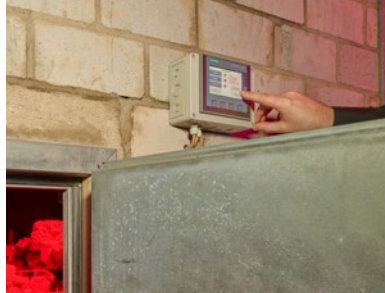
Along the tour route are two Simatic HMI KTP400 Basic Panels used to control permanently installed light and sound effects (left). The heart of the whole installation is the control cabinet, which, thanks to the compact design of Simatic S7-1200, could be completely retained (above)
