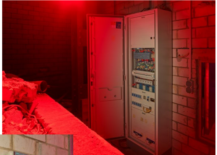
Along the tour route are two Simatic HMI KTP400 Basic Panels used to control permanently installed light and sound effects (left). The heart of the whole installation is the control cabinet, which, thanks to the compact design of Simatic S7-1200, could be completely retained (above)
