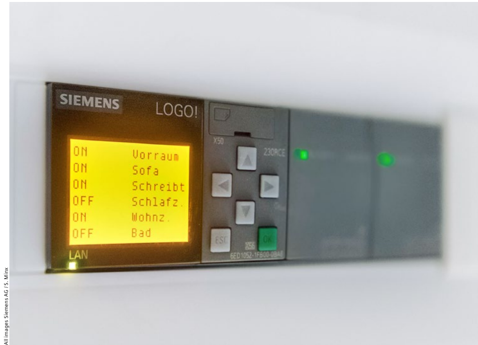
The LOGO! logic module controls the lights, ambient temperature, blinds, access controls, and other functions in the Hotel Bayerischer Hof
