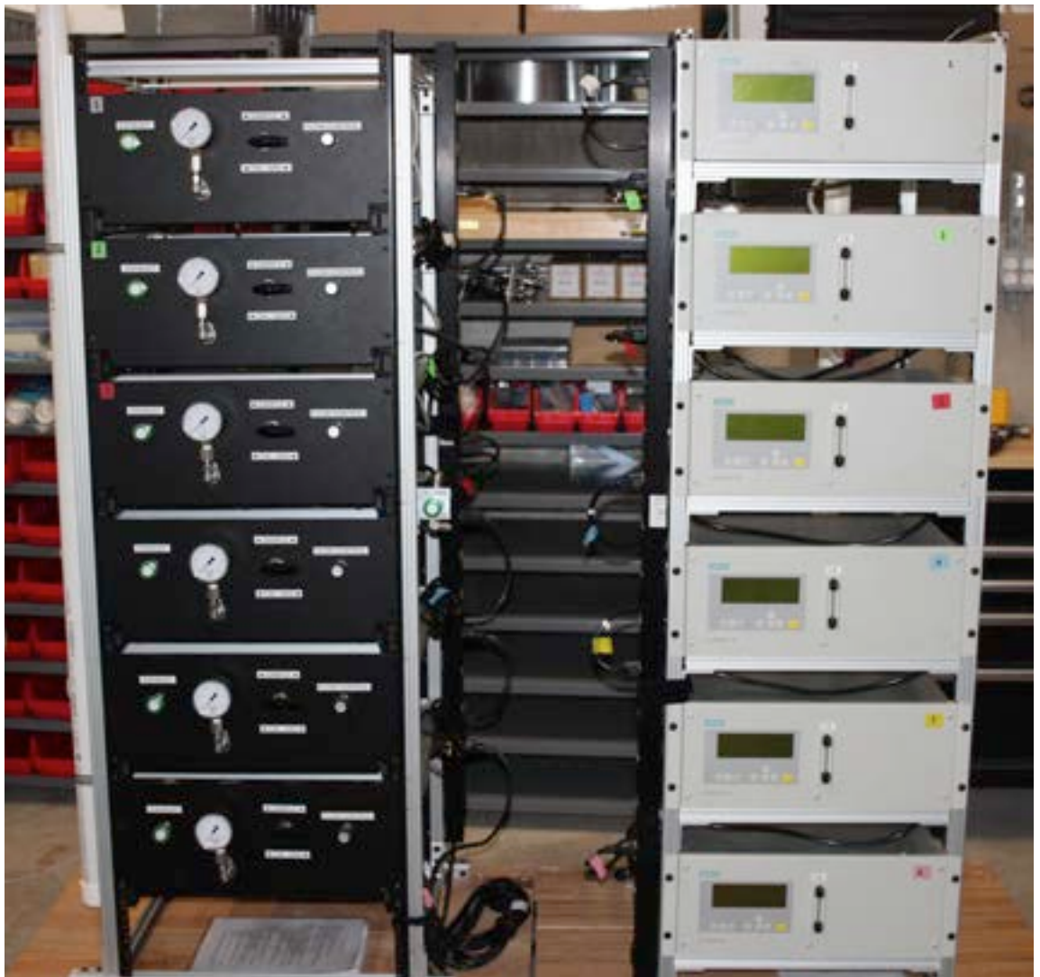
Rack of ULTRAMAT 23 with sample conditioning system in real-life scenario.
